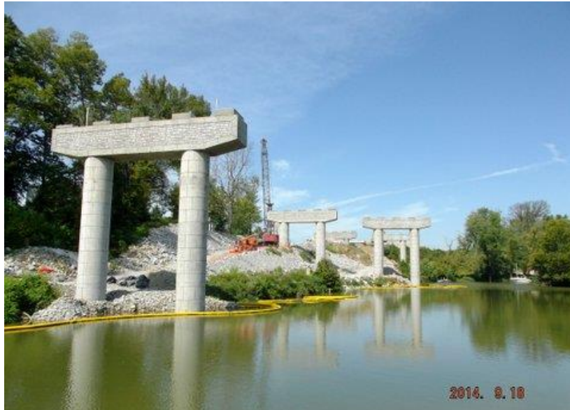
East End - Harrods Creek Construction
