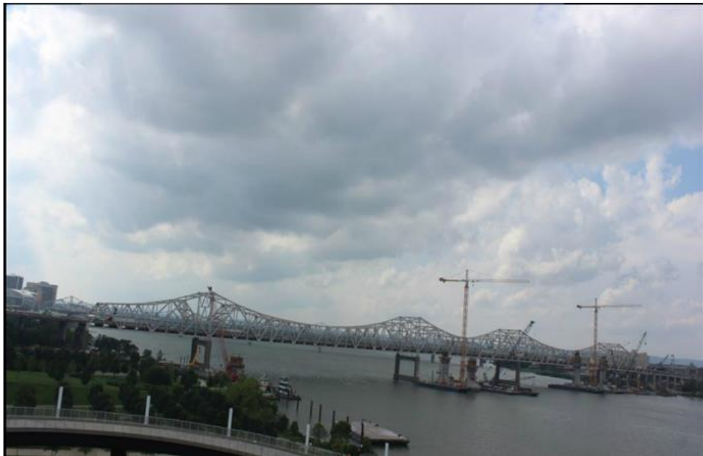
Downtown Crossing – New Ohio River Bridge Construction
