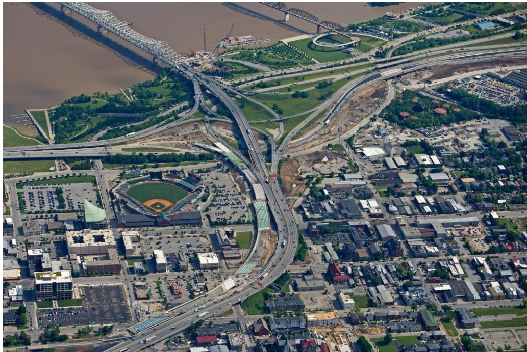
Kennedy Interchange Construction - 2014
