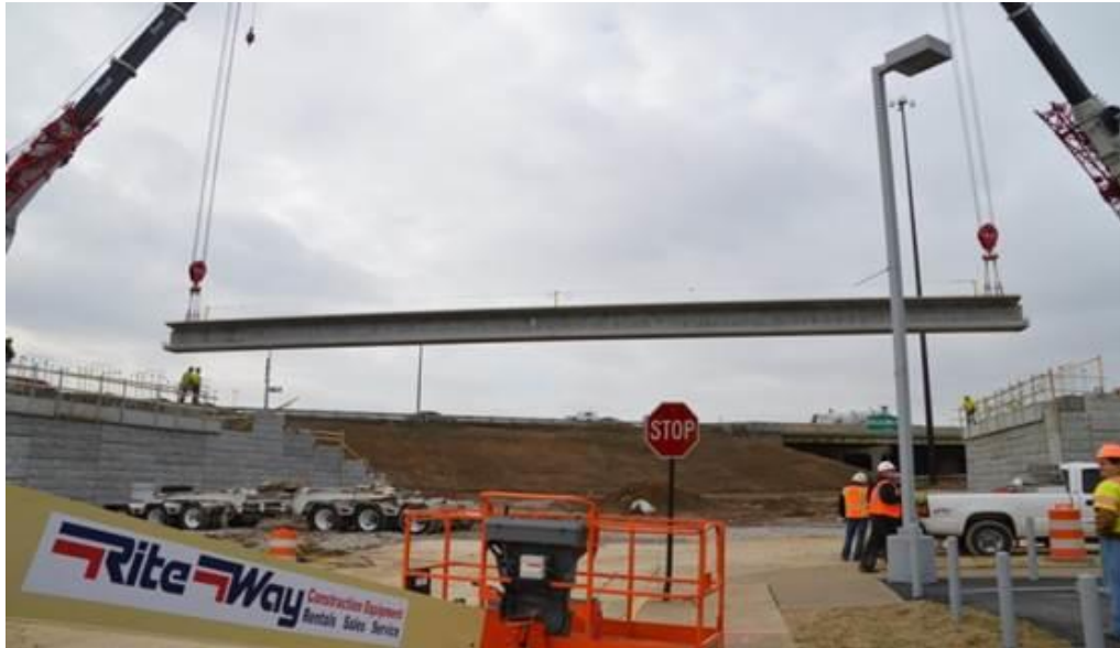
Downtown Crossing – Beam setting in Indiana
