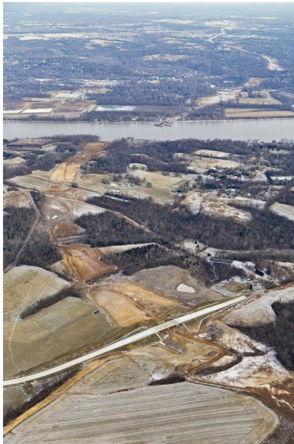
East End Crossing Construction
