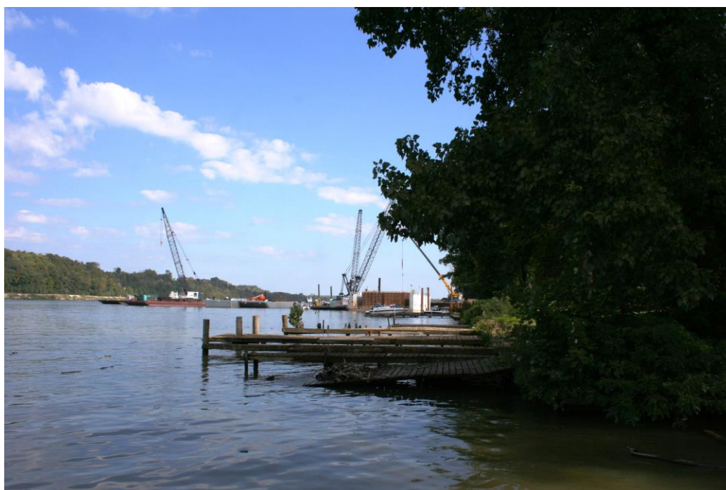
East End Bridge Construction
