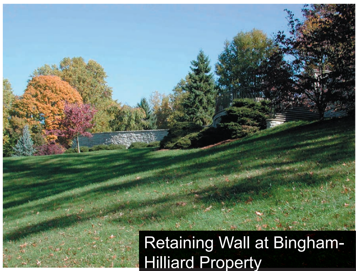
Retaining Wall at Bingham-Hilliard Property
