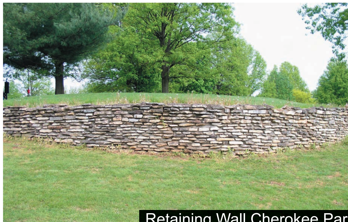
Retaining Wall Cherokee Park
