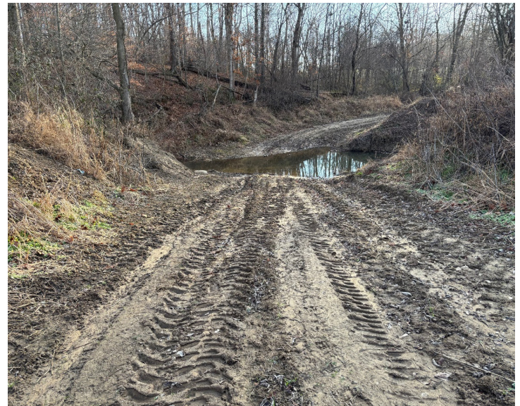
This permanent agricultural crossing was also used for a timber harvest. There is no hardening or diversions, and a lot of loose soil will go directly into a perennial stream. Photo by Jennifer Sobecki, DNR
