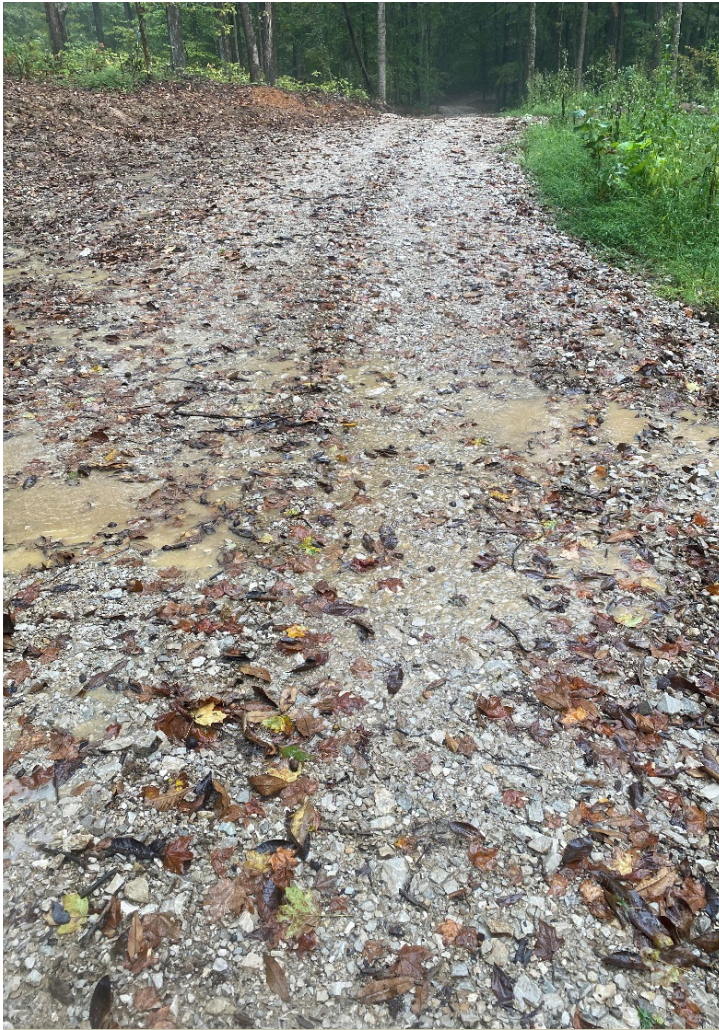
An outslope on this access road channels runoff to the forest floor. This prevents runoff from continuing down the access road, thus limiting erosion potential. Photo by Duane McCoy, DNR
