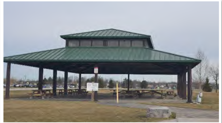
Large Accessible Shelter House Pavilion
