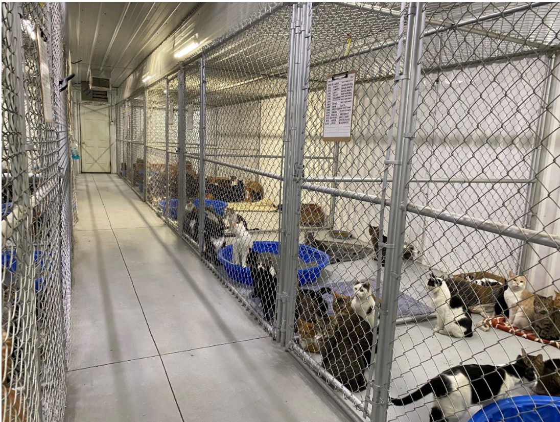
IMG 6723 VBB, 12-27-23, cat facility Room 3
