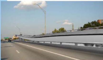
View from I-65 Northbound
