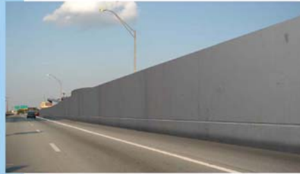
View from I-65 Northbound
