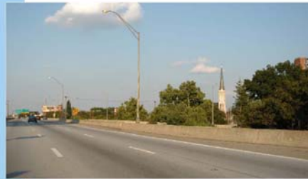
View from I-65 Northbound
