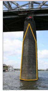
2 nd Street Bridge Pier
