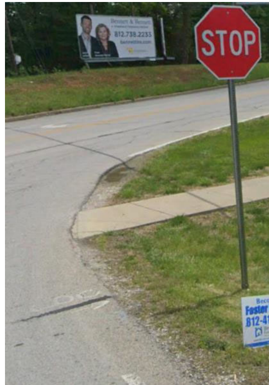
Curb ramp at IN-337 with no DW (Source: Google Earth Streetview)
