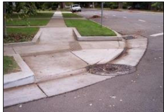
Example combination curb ramp, with a perpendicular ramp to a common landing and adjacent parallel ramps.
