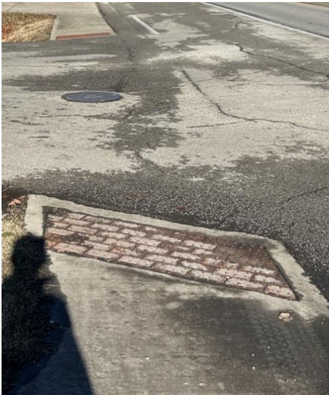
Curb ramps at Wyandotte Avenue, including one with brick paver DW
