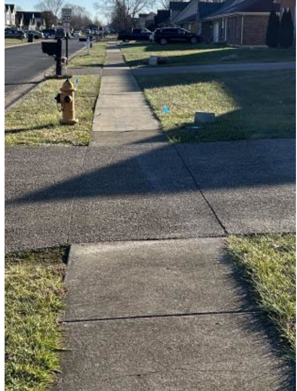
Typical driveway crossing at PAR
