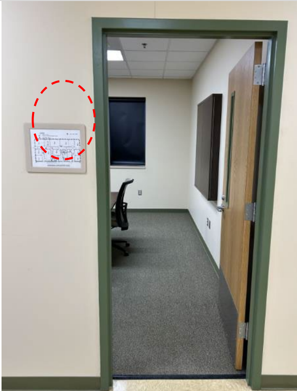
Item #36 Entry door with no signage
