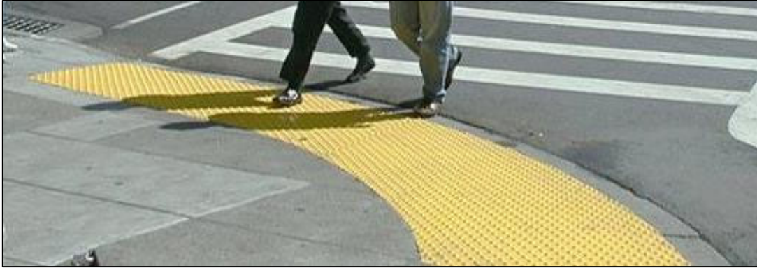
Diagonal blended transition/depressed corner. Note the level transition from the street crossing to the PAR.
