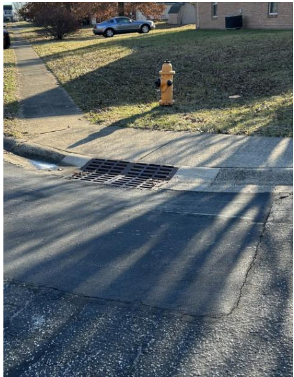
Curb ramp at SE quadrant of Settlers Trace & Liberty Way with drain structure in ramp (typical also at Frontier Ct. and Colonial Way)
