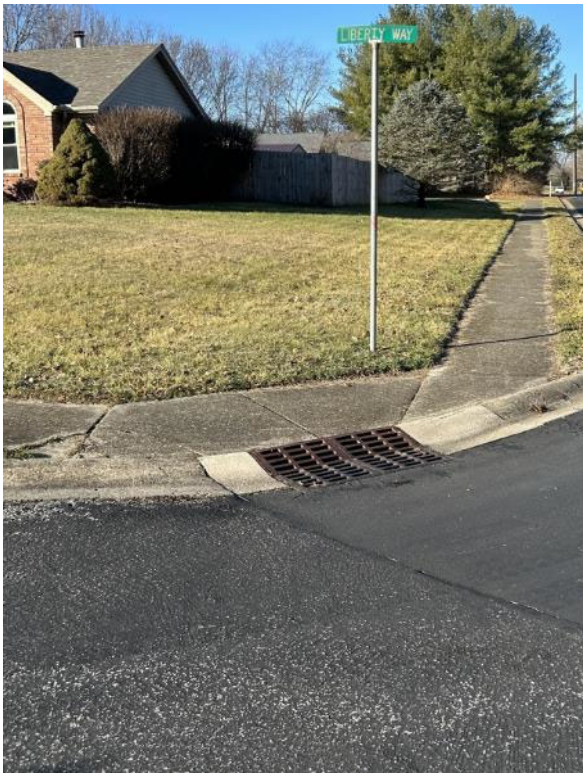
Curb ramp at SW quadrant of Settlers Trace & Liberty Way with drain structure in ramp (typical also at Frontier Ct. and Colonial Way)
