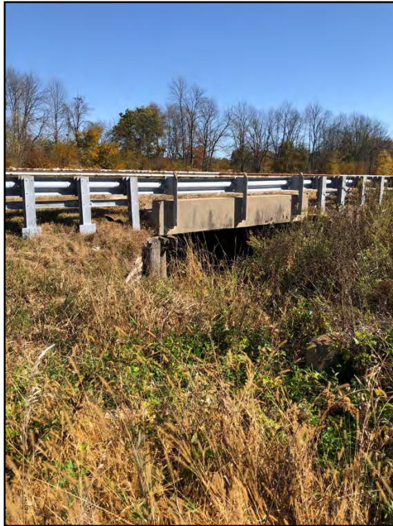
Photo 9: Looking at UNT to Sand Branch with a view of the west side of the project small structure.
