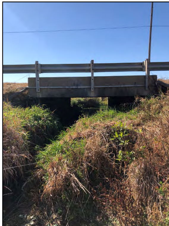
Photo 8: Looking at UNT to Sand Branch with a view of the east side of the project small structure.
