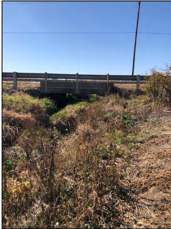
Photo 7: Looking at UNT to Sand Branch with a view of the east side of the project small structure.
