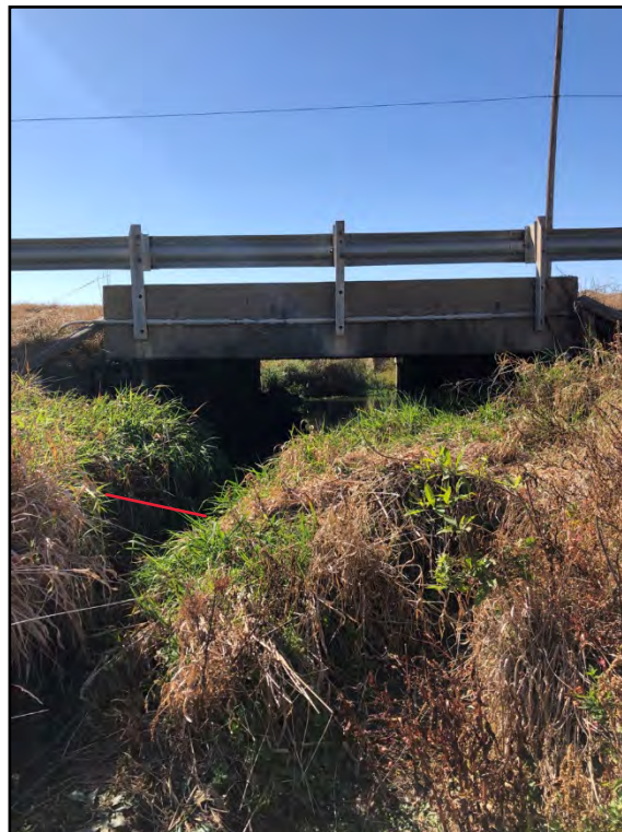
Photo 8: Looking west at UNT to Sand Branch with a view of the east side of the project small structure.
