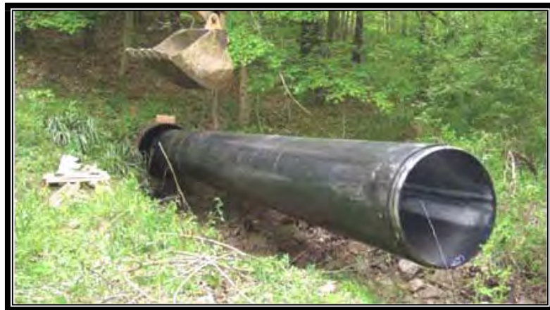
Figure 6-4. Pulling Pipe Liner
