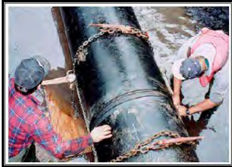
Figure 6-3. Jointing a Liner
