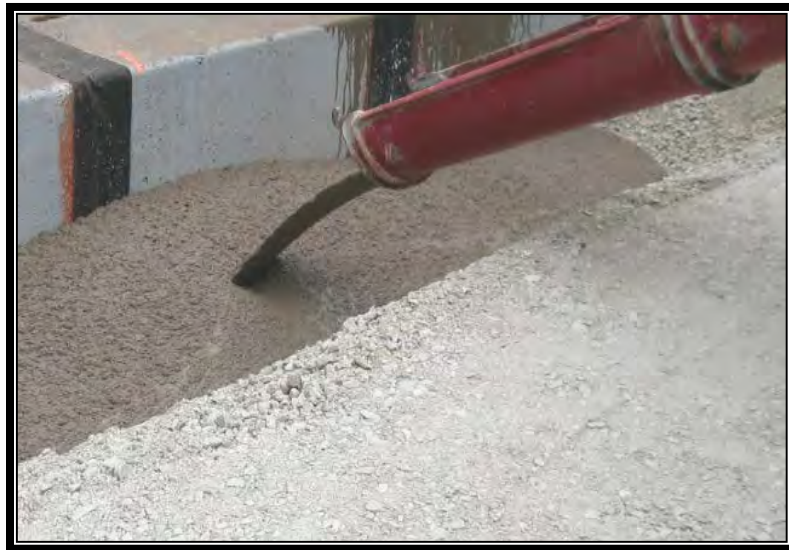
Figure 5-1. Flowable Backfill for Box Structure
