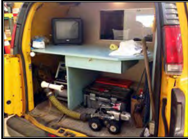
Figure 5-4. Van with Video Inspection Equipment
