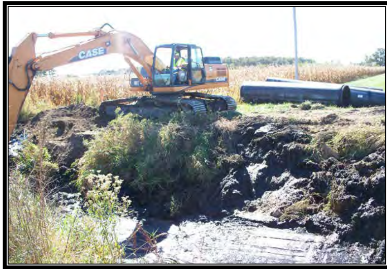
Figure 2-2. Removing Unsuitable Material
