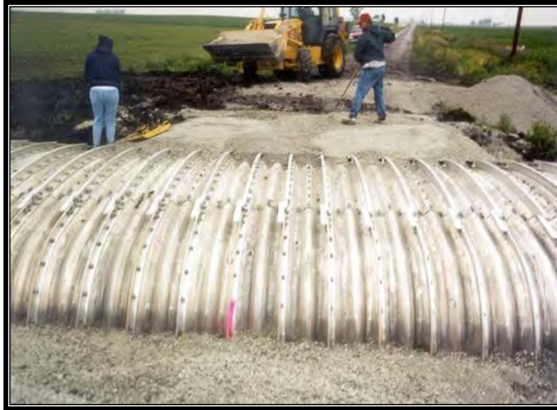
Figure 5-2. Structural Backfill
