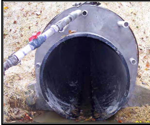
Figure 6-6. Grouting Pipe Liner
