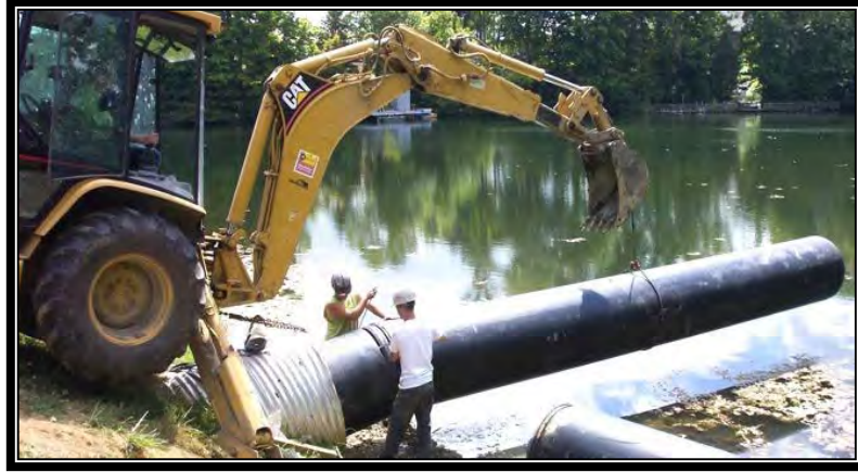
Figure 6-5. Pushing Pipe Liner over Water
