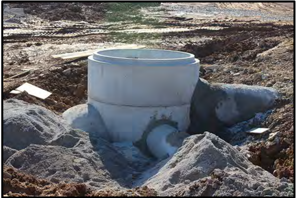
Figure 4-3 Manhole with Concrete Collar Connections
