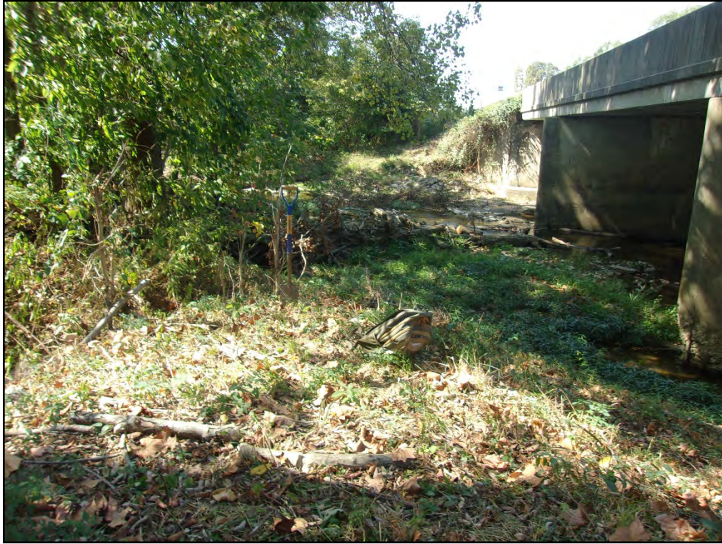
Photo 13: Looking west at SP2.
