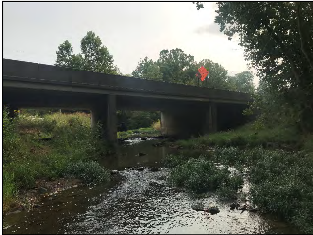
Photo 11: Looking northeast at US 50 Bridge over Six Mile Creek.
