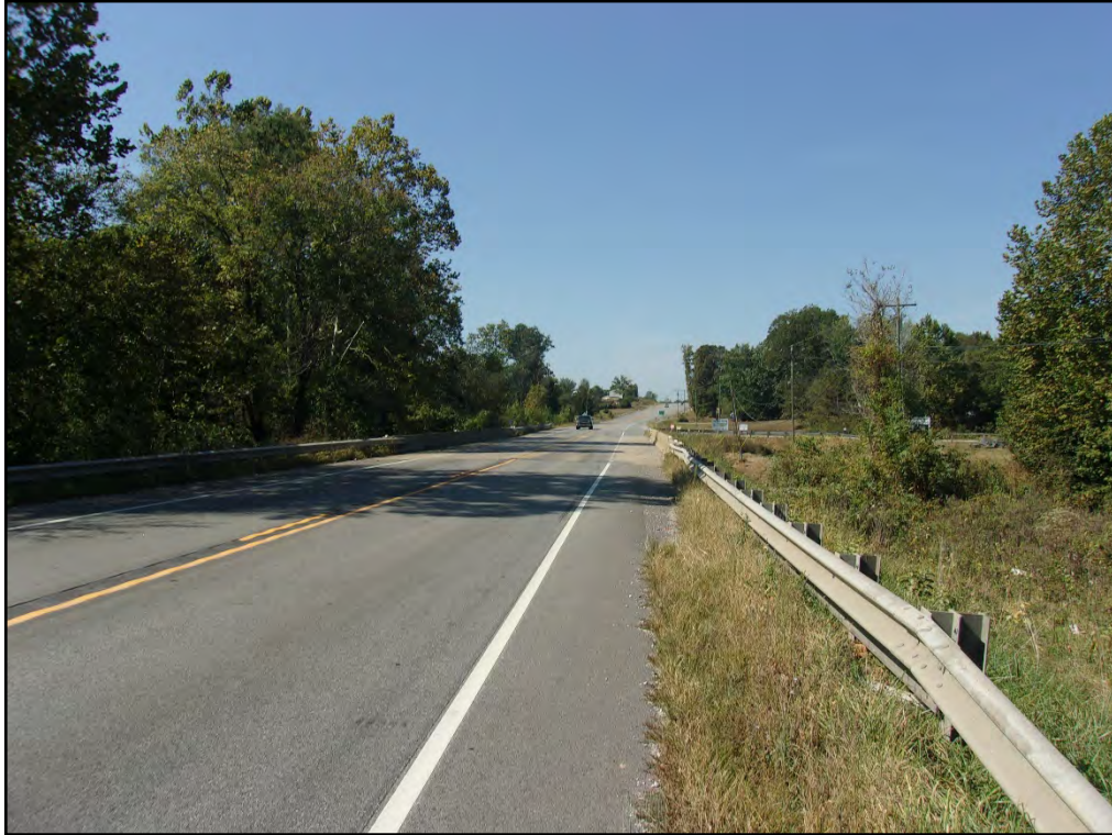
Photo 1: Looking west along US 50 from near east end of project area.
