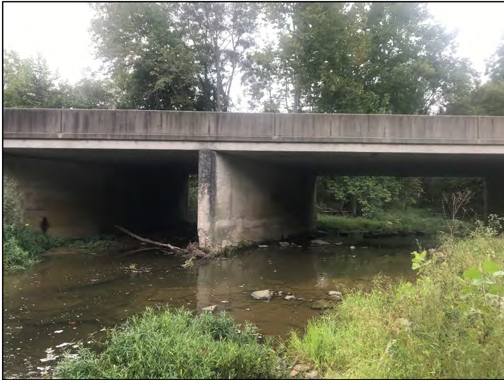
Photo 17: Looking south, downstream, at US 50 Bridge over Six Mile Creek.
