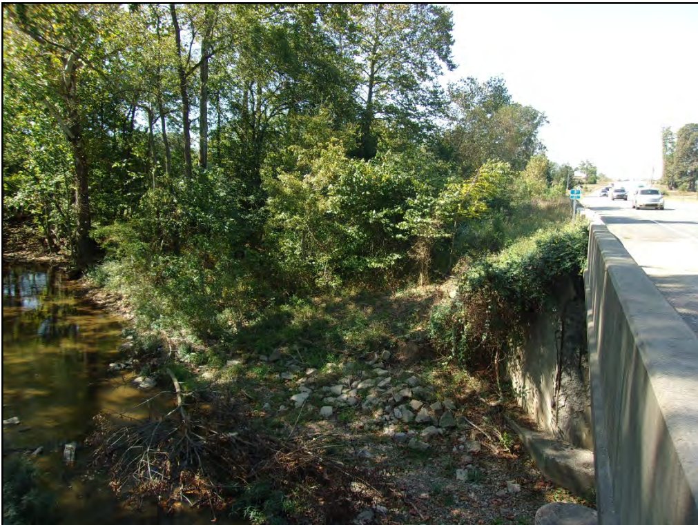
Photo 10: Looking at southwest quadrant from bridge.
