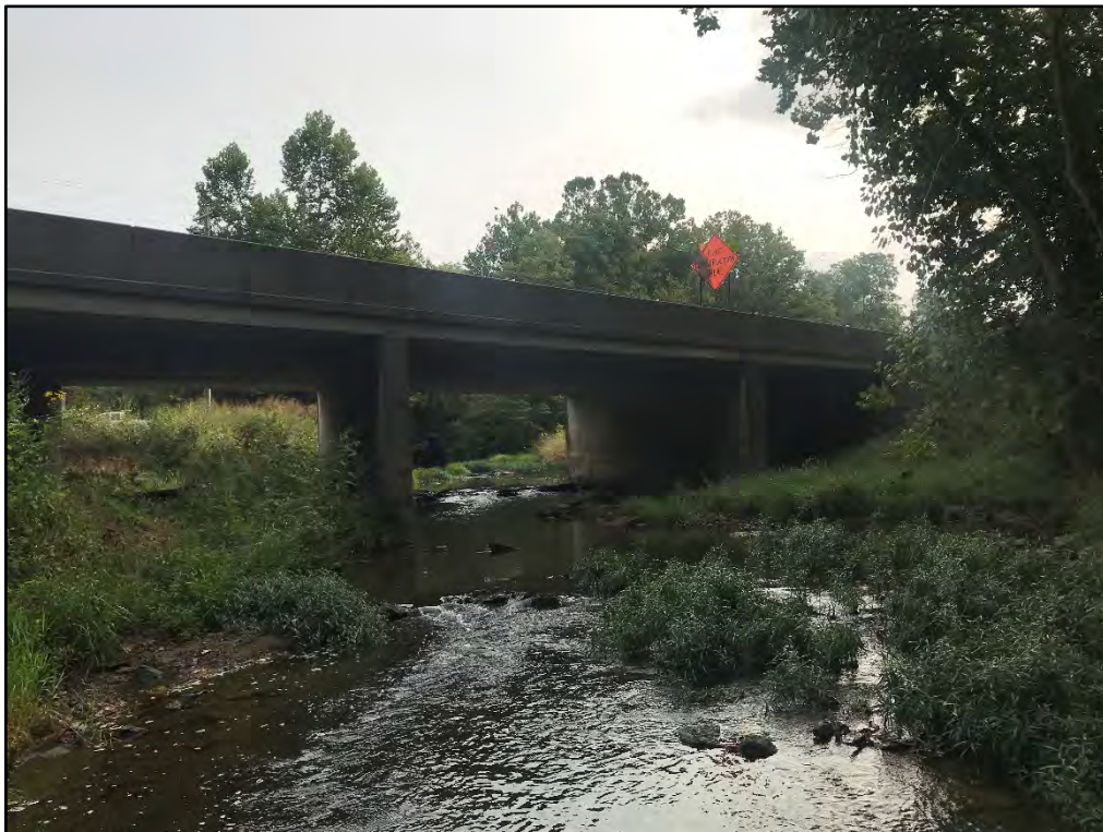
Photo 18 Looking north, upstream, at US 50 Bridge over Six Mile Creek
