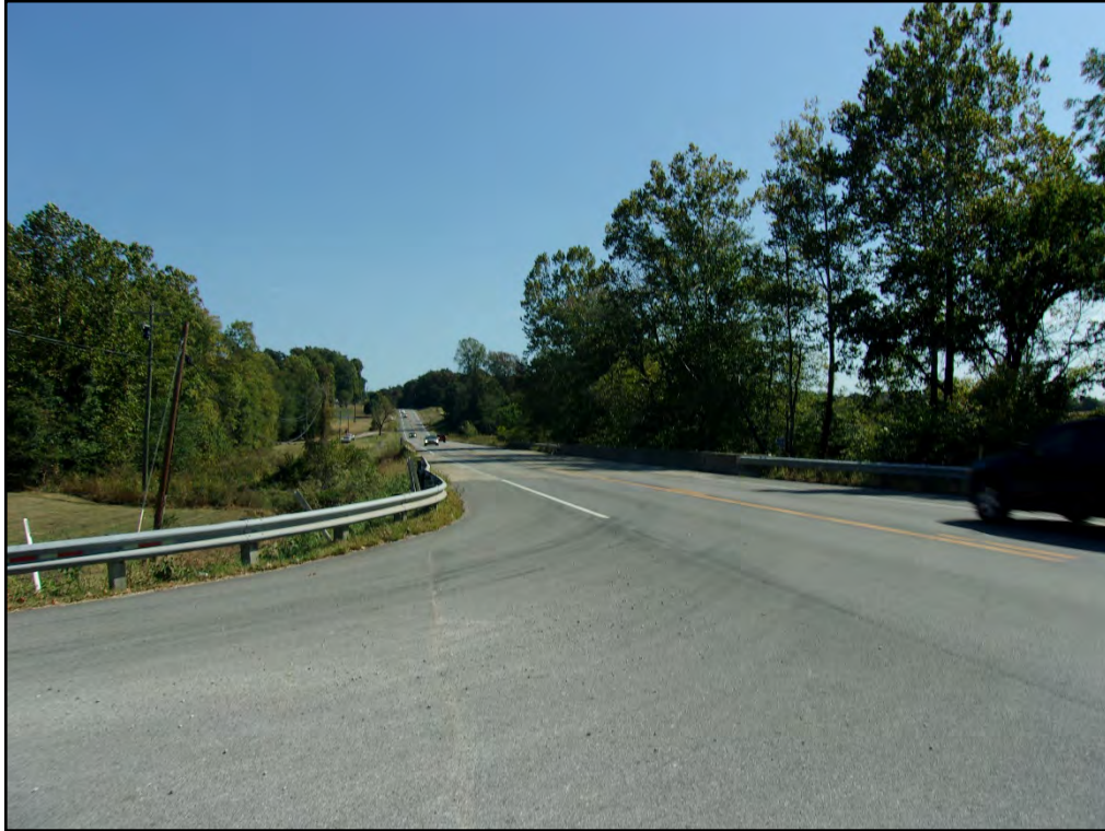
Photo 3: Looking east along US 50 from intersection with Washington Street.
