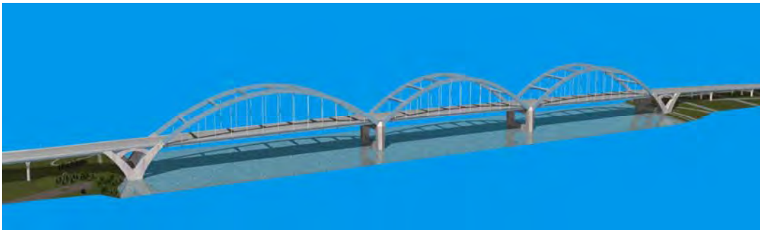
Alternative 3: Three Span Thru Arch
