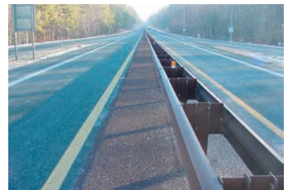
MD 90 coated steel W-beam.
