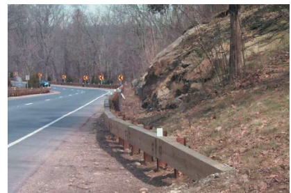
Merritt Parkway timber guardrail.
