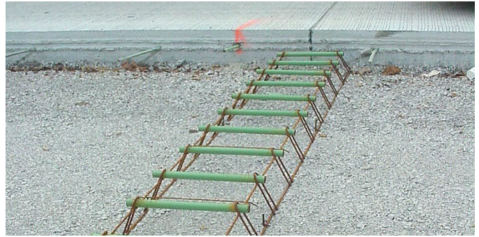
Figure 7-3 Tie Bar Adjustment at Dowel Bar Assembly
