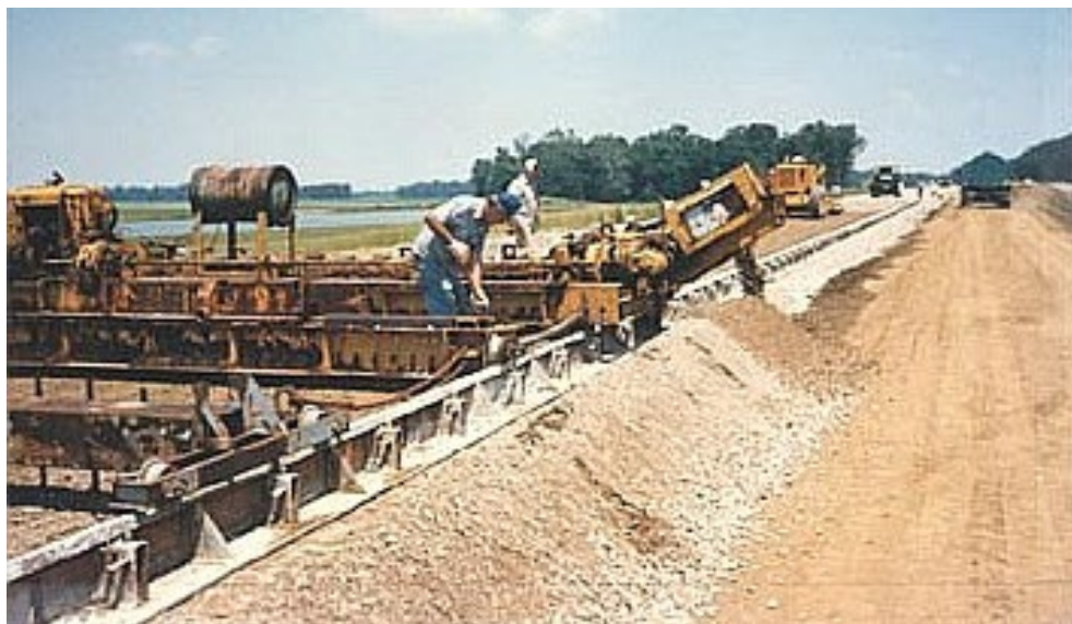
Figure 2-1 Form Paving Spreader
