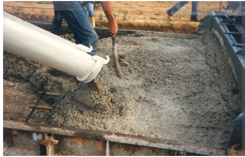
Figure 4-10 Handheld Vibrator
