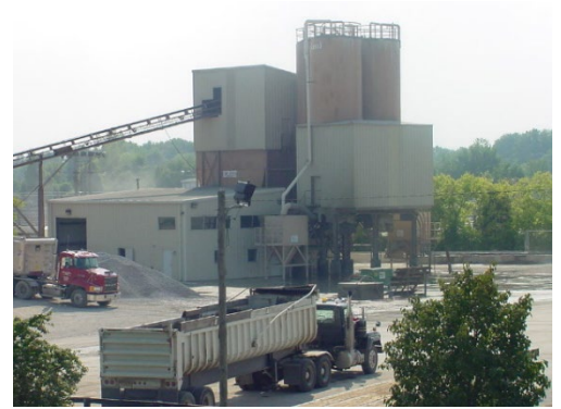
Figure 4-2 Ready Mix Plant
