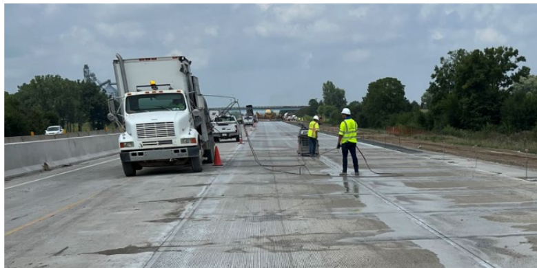
Figure 4-11 Sawing joints into concrete
