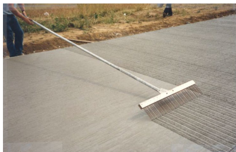
Figure 4-9 Steel Tine Hand Tool
