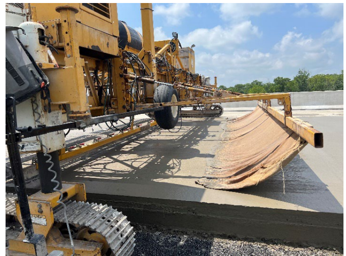
Figure 4-7 Tining Equipment
