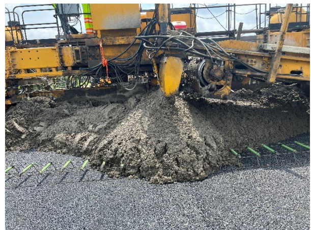
Figure 4-6 Slip-Form Paver
