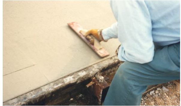
Figure 6-7 Hand Finishing
