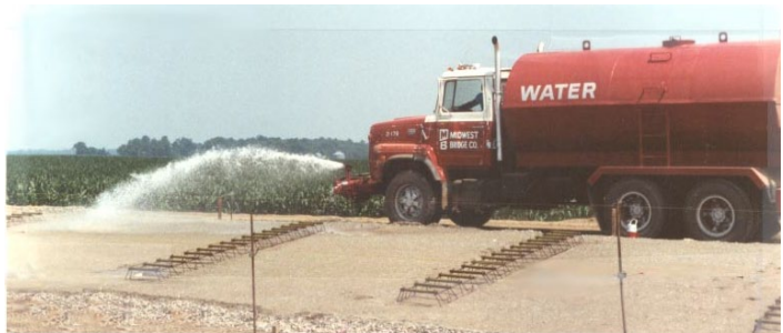
Figure 6-1 Subbase Watering
