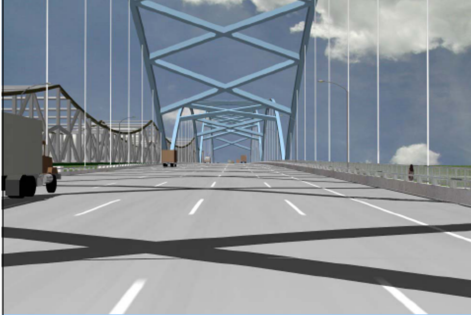
ALTERNATIVE 1: THREE SPAN TIED ARCH
