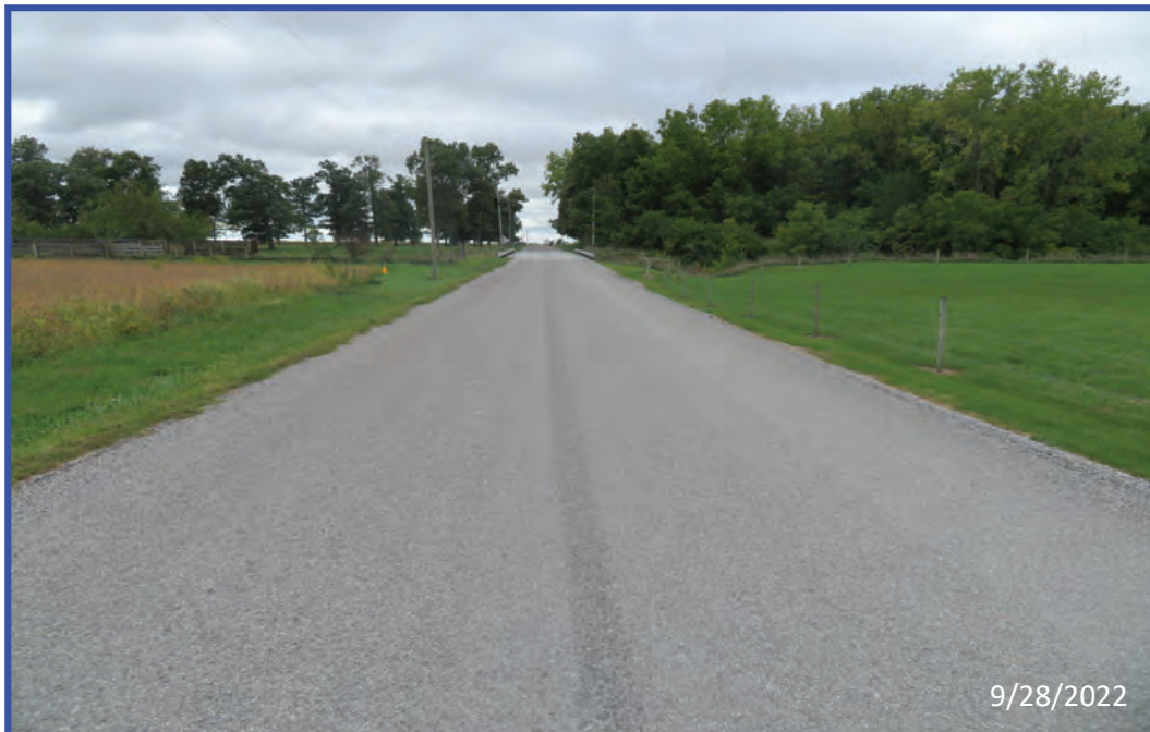
10) Looking south along CR 100 East towards Bridge No. 180
