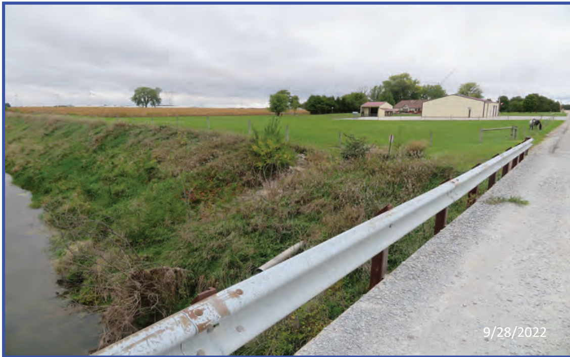
5) Looking northwest at the northwest quadrant of Bridge No. 180
