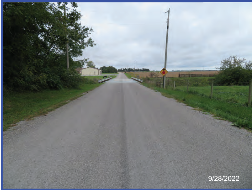
9) Looking north along CR 100 East towards Bridge No. 180
