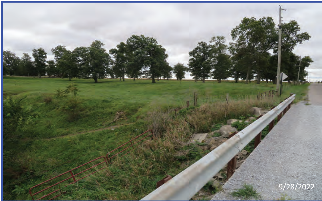
4) Looking southeast at the southeast quadrant of Bridge No. 180
