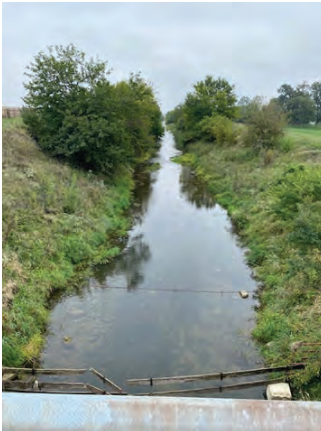
Photograph # 5 on the bridge, looking east downstream
