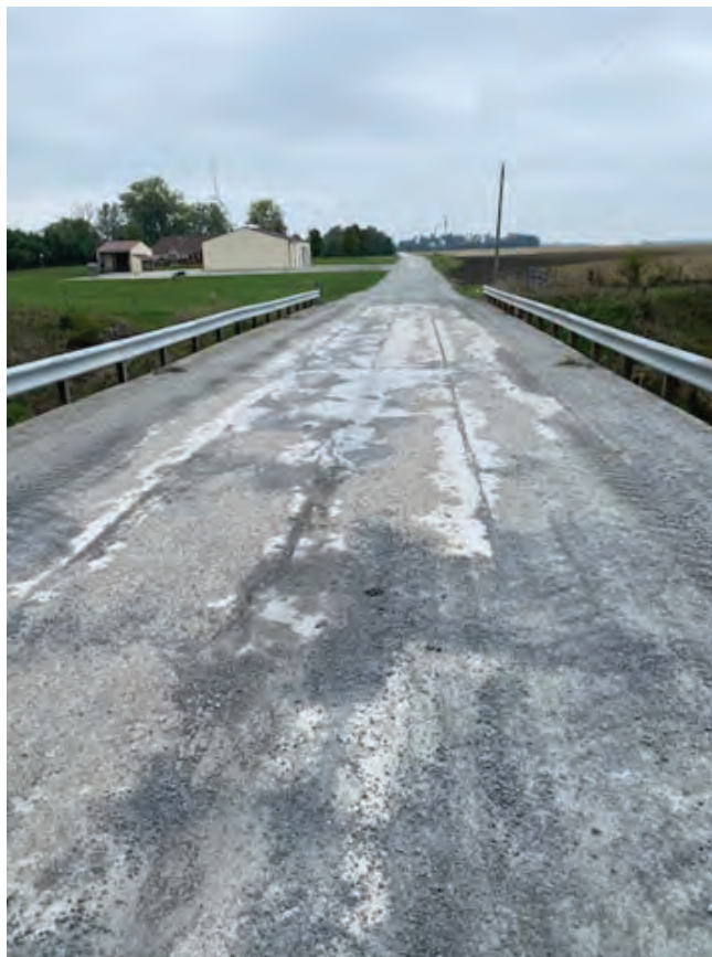
Photograph # 2 south end of bridge, looking north
