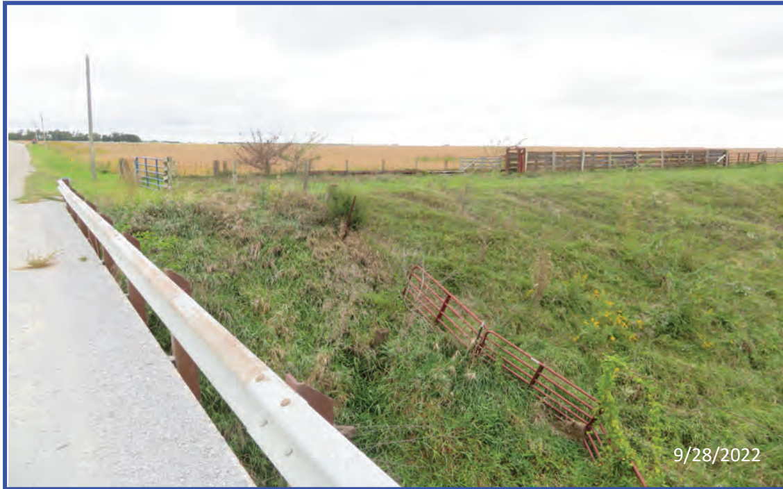
3) Looking northeast at the northeast quadrant of Bridge No. 180
