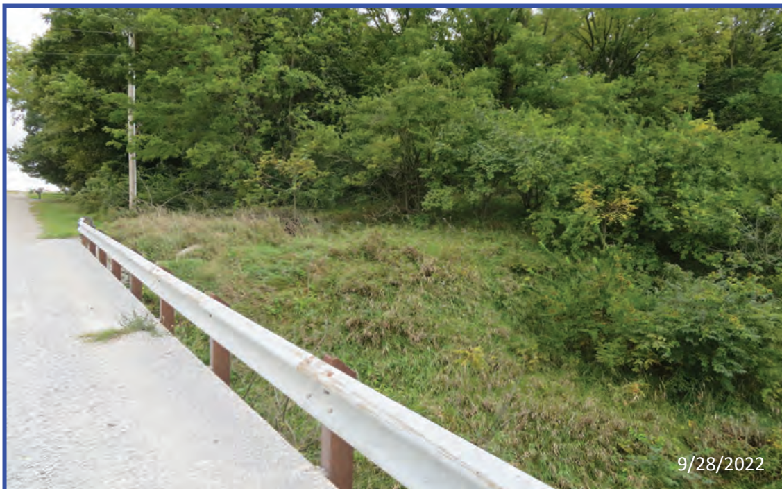
6) Looking southwest at the southwest quadrant of Bridge No. 180
