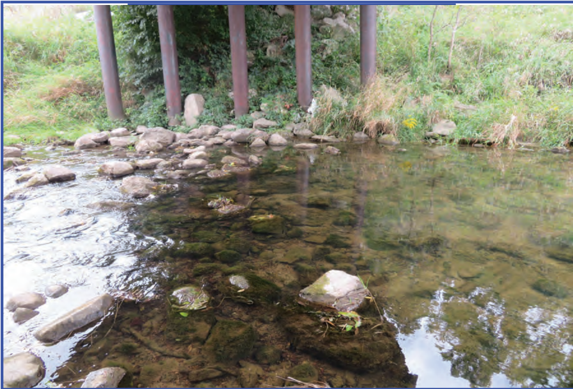
7) Looking north across Big Creek at riffle under Bridge No. 180
