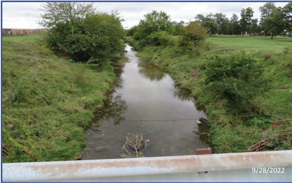
1) Looking east (downstream) along Big Creek from Bridge No. 180
