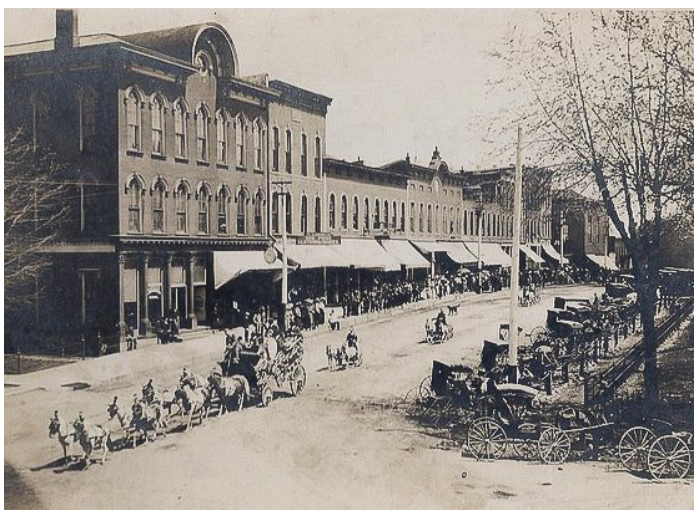
1900s Parade, Source: Parke County Covered Bridge Festival
