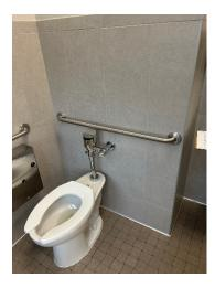
Wall width too short to allow needed spacing for grab bar
