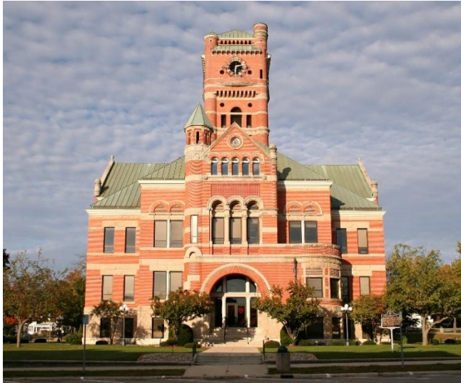
Figure 4: Noble County Courthouse
