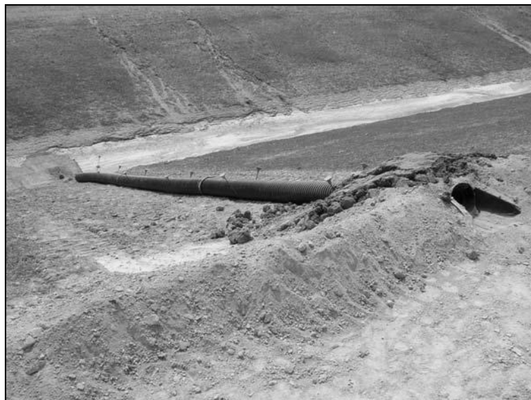
Figure 1: Temporary Slope Drain with Flared-End Section
