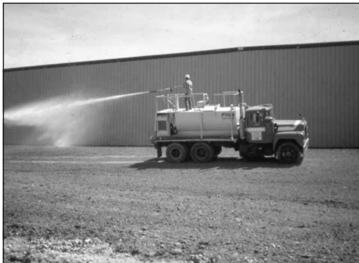
Figure 3: Hydroseeding
