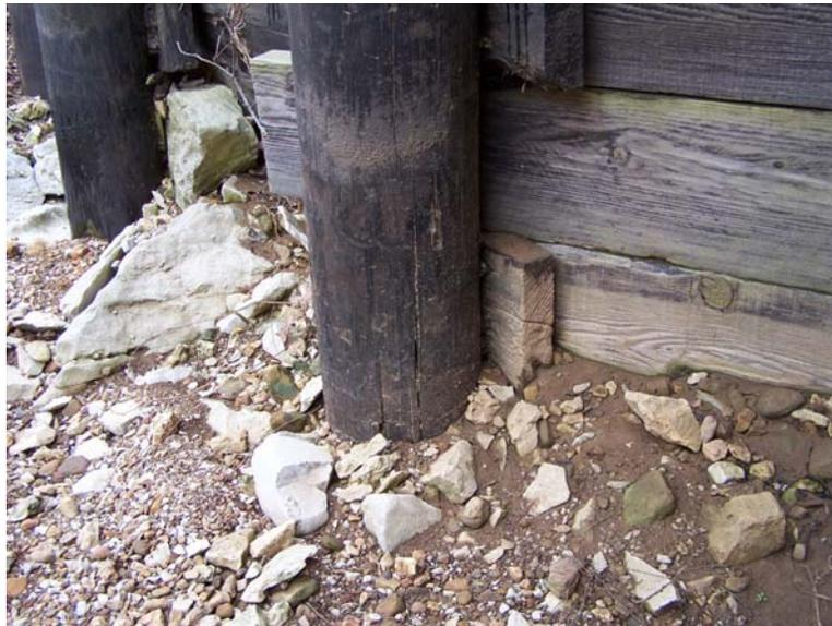
Looking south at rotten pile at east end of south bent
