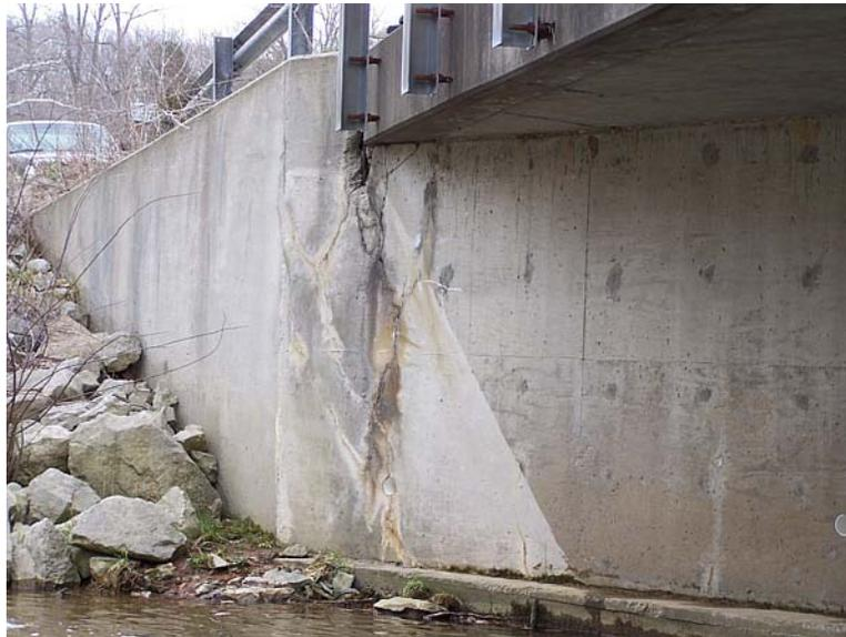
Looking south at cracks in abutment at southeast corner
