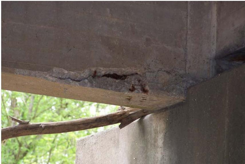
Looking northeasterly at crack and spall in bottom of Girder #1
