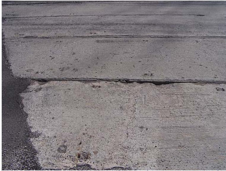
Looking easterly at hairline transverse cracks in north beam ends
