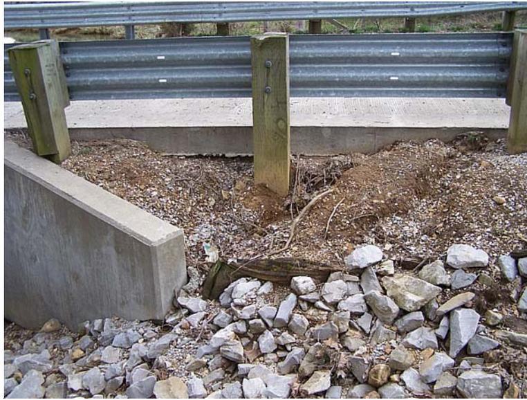
Looking south at erosion and undermined west approach slab
