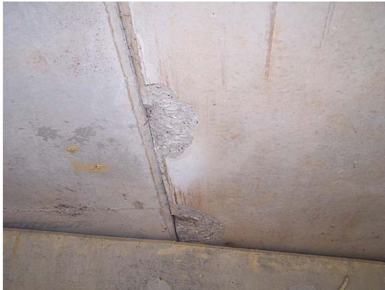
Looking north at spalls on bottom of middle beam at the north end
