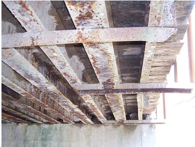
Looking north at bent channel on east side and heavy rust on steel
