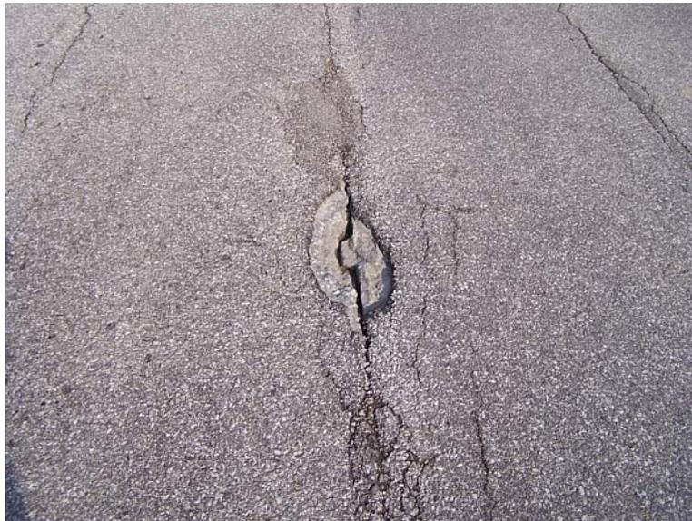
Looking northwest at cracked wearing surface over beam joints
