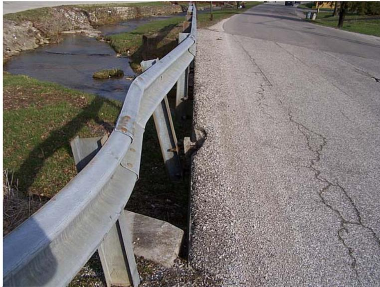
Looking northwesterly at collision damage to railing with posts knocked loose and spalls in coping at southwest corner
