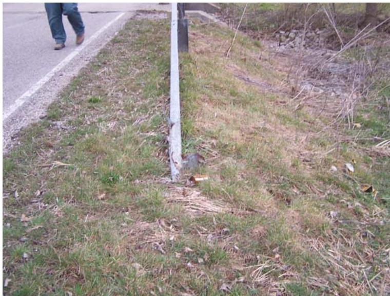
Looking westerly at damaged guardrail in northeast quadrant
