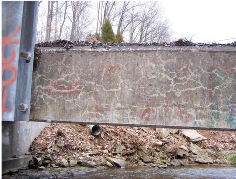
Looking north at extensive cracking of south coping
