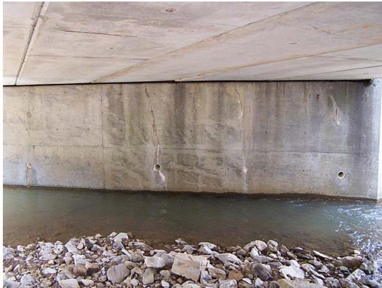
Looking north at cracks in north abutment
