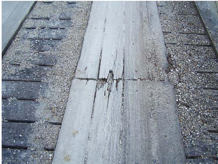
Looking north at rotting runners on east side
