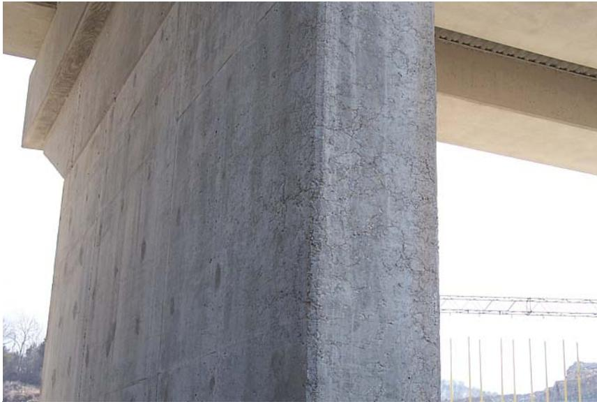
Looking northerly at honeycombed concrete in south end of west pier
