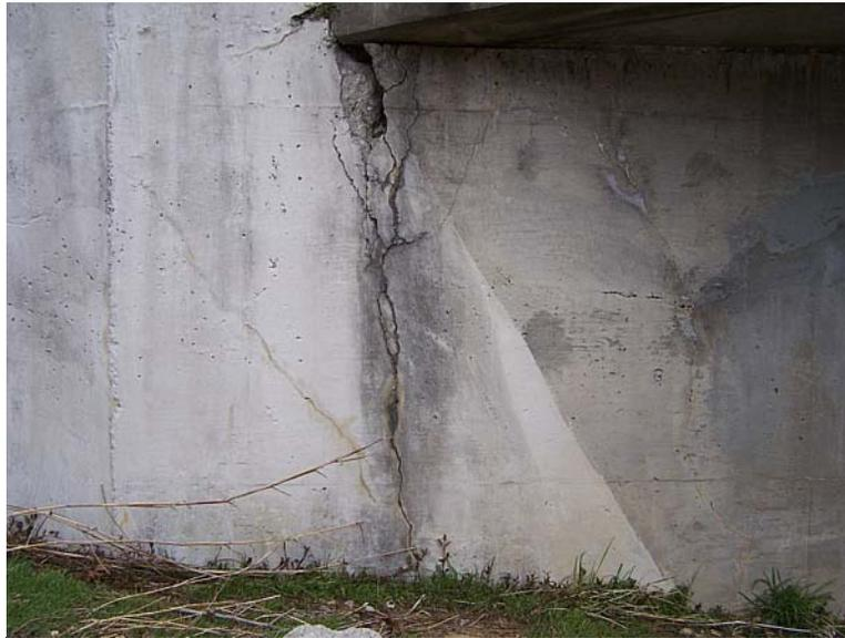
Looking north at cracks in abutment at northwest corner
