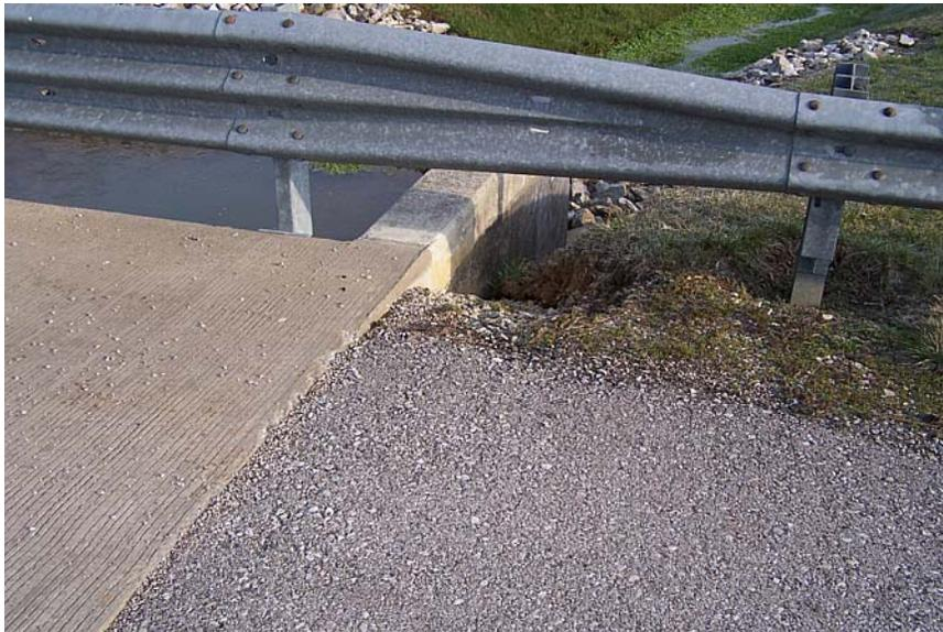
Looking north at shoulder erosion at northeast wing
