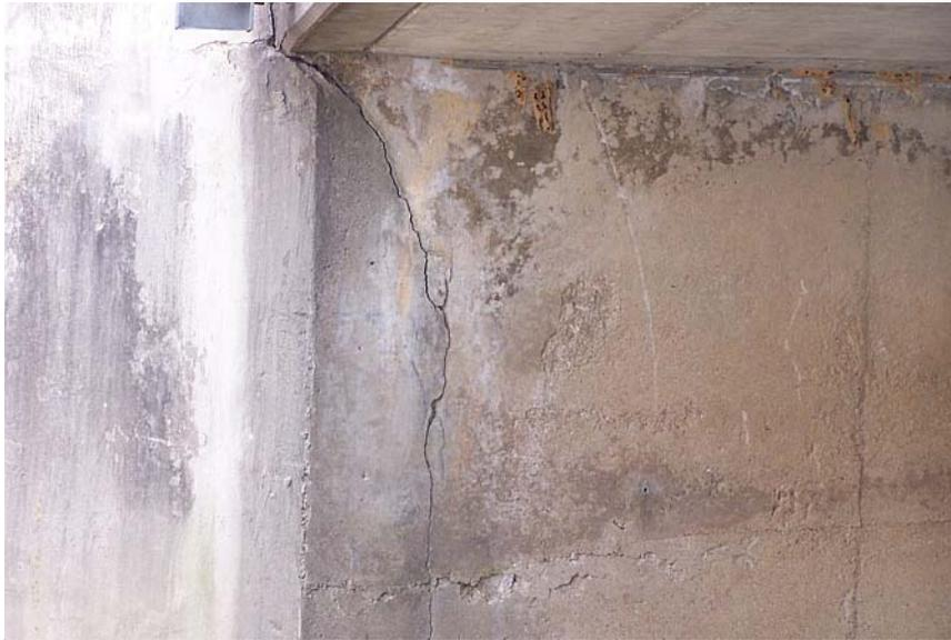
Looking northerly at crack in abutment at northwest corner
