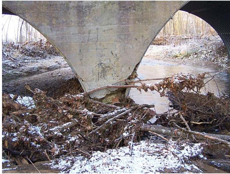
Looking southwesterly at drift and spalled concrete between spans
