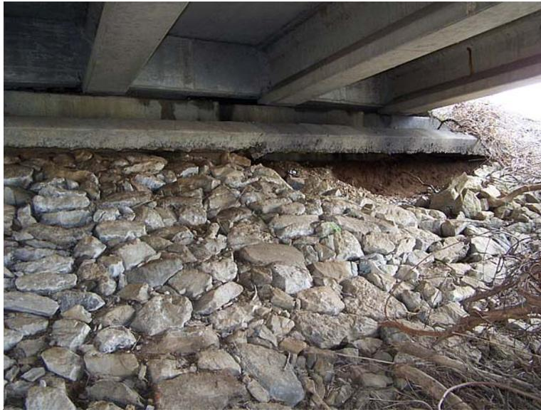
Looking northeast at north slopewall erosion and settlement
