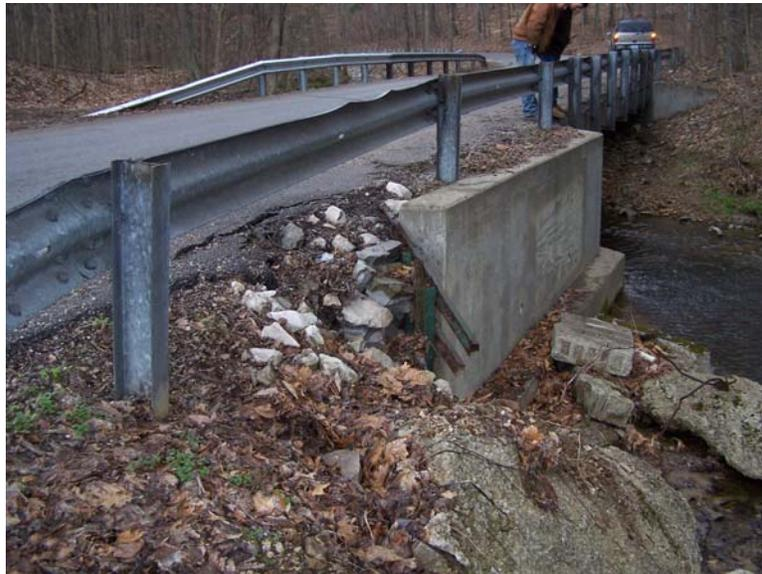
Looking northerly at erosion and debris around southeast wing
