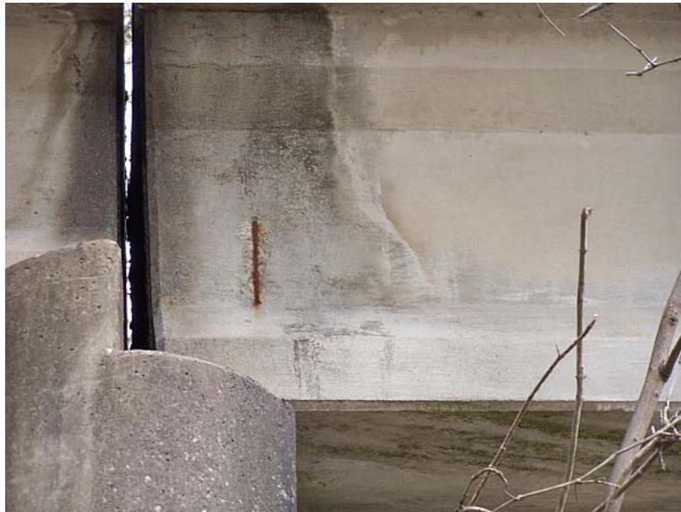
Looking east at beam spall over west end of north pier
