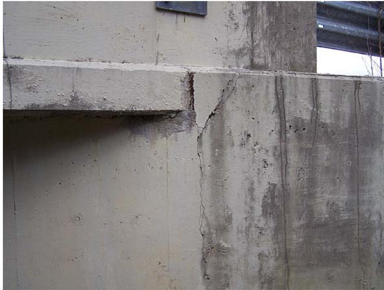
Looking northwesterly at cracks and spalls at northeast corner
