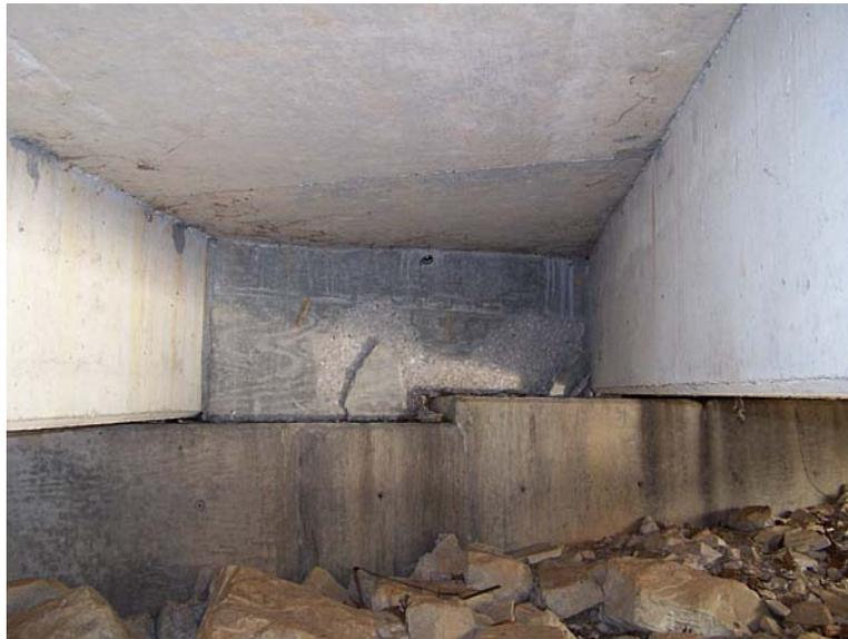
Looking northerly at spalled diaphragm over north bent
