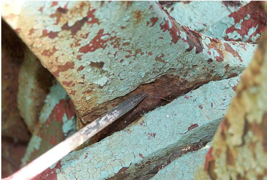
Looking northerly at section loss on inside vertical member U2-L3 in north truss
