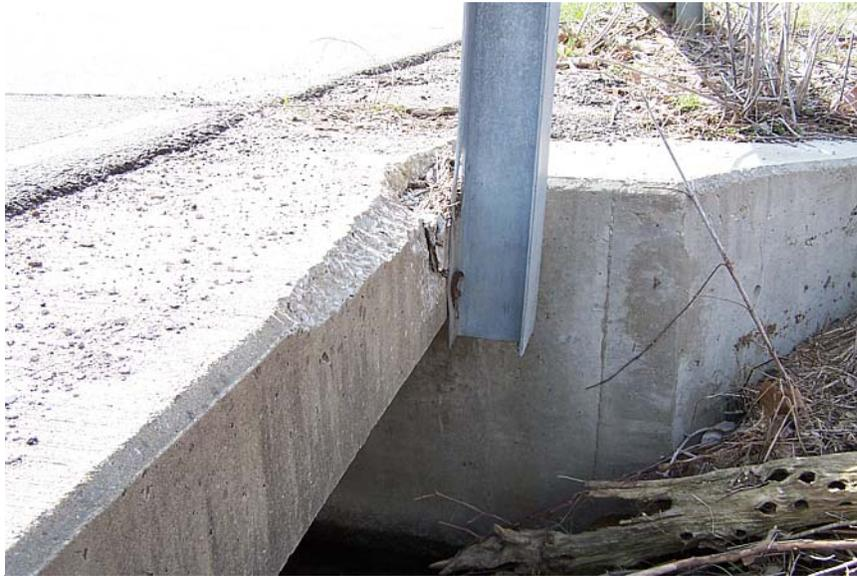
Looking southerly at beam spall in southwest corner caused by railing collision which knocked loose railing post
