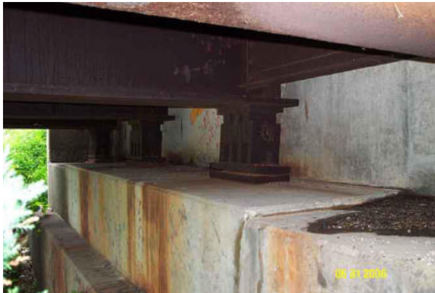
Bearings at northwest corner
