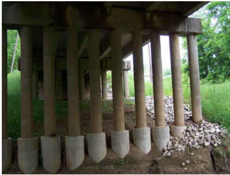
Addition concrete encasement of piles at Pier No.3
