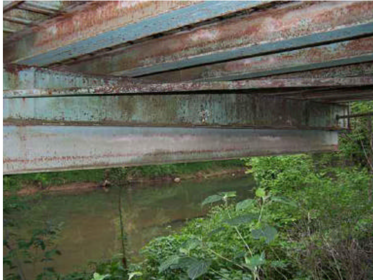
Addition beam welded to bottom of floor beam
