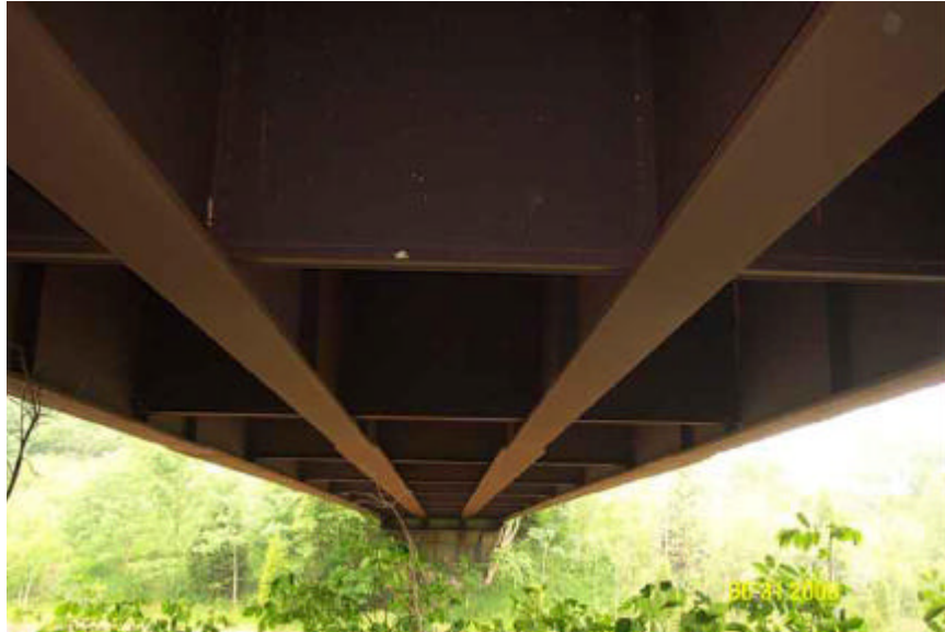
Underside of bridge looking south
