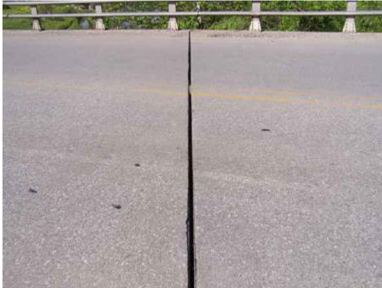
Open joint over south pier
