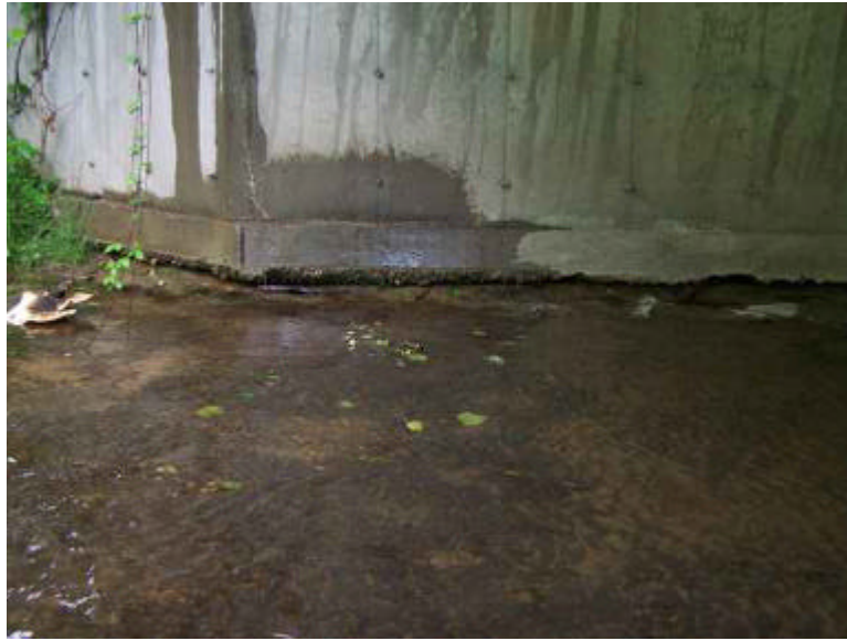
West abutment set on rock
