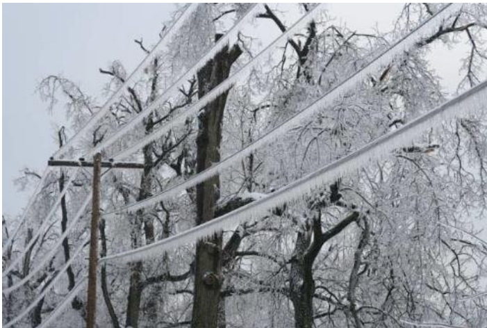
Figure 3-19 Ice Covered Power Lines
