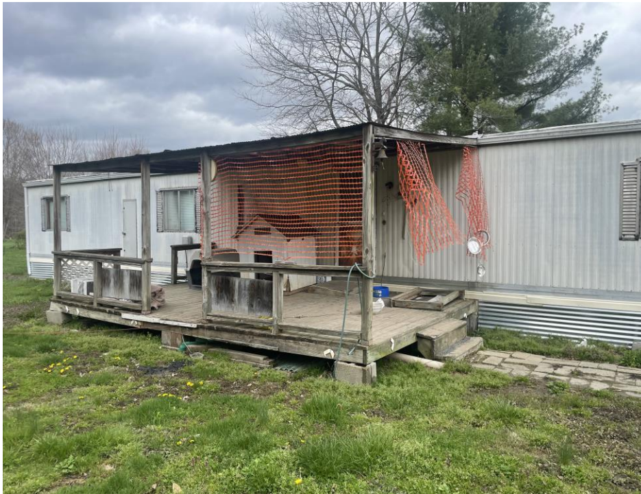
View from the Eastern front of the home.
