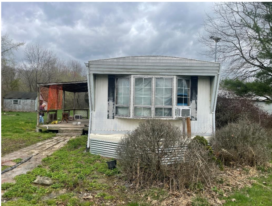
View from the East side of the home.
