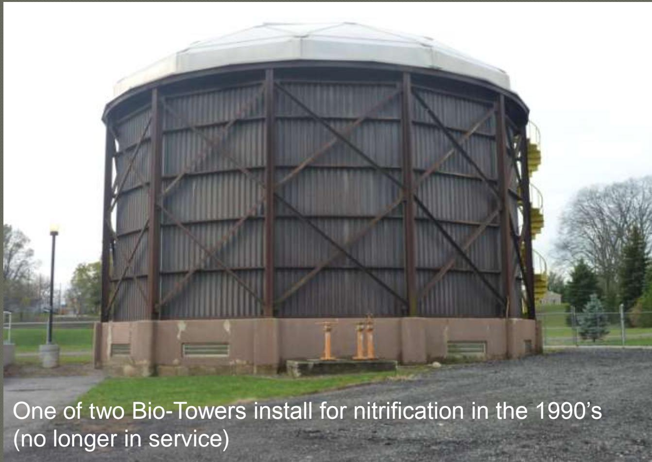
One of two Bio-Towers install for nitrification in the 1990's
