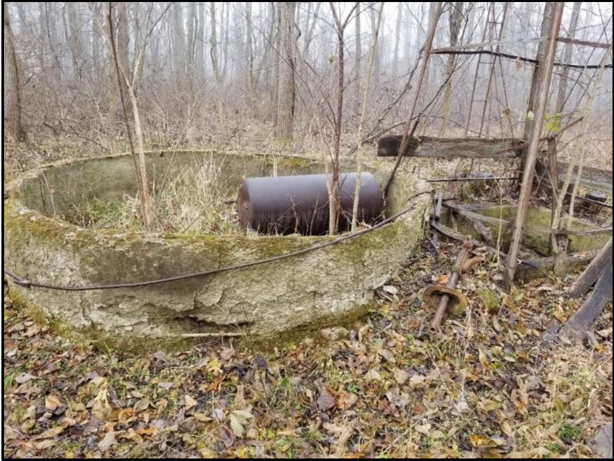
Figure 11. Water storage tank foundation feature at site 12MY711 (Photo by Sean Coughlin, Ball State University).
