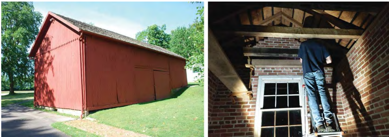
Figure 7. Huddleston carriage house's north eave façade and east gable façade (left). Interior sampling of the smokehouse's frame roof (right) (Photo credit: Christopher Baas).
