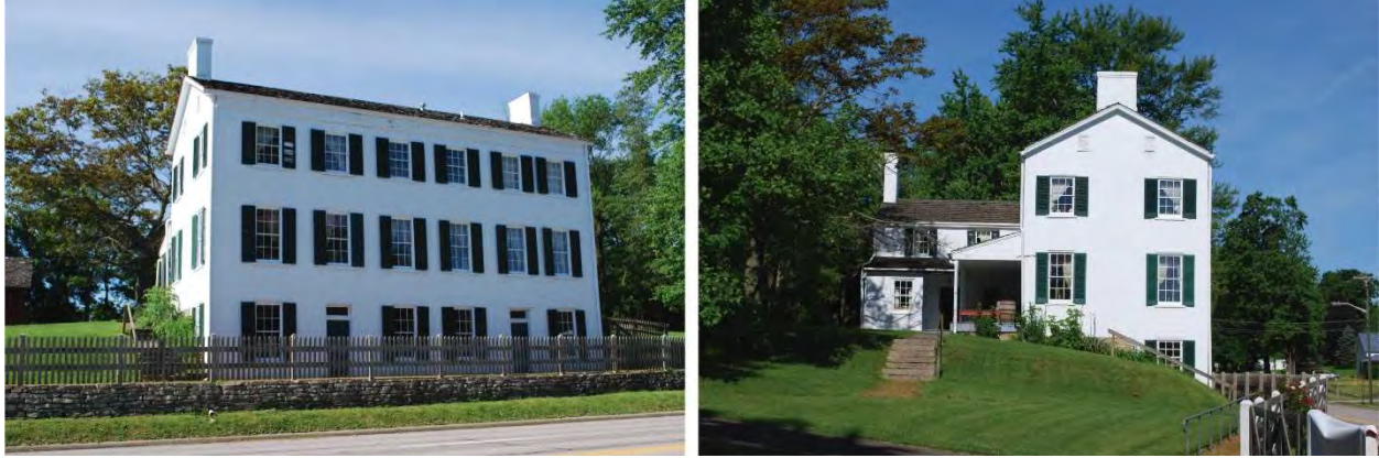
Figure 4. Huddleston house's north façade (left) and gable end east façade (right). The house is constructed into a hill that provides National Road access to the cellar and 1 st story access to the house from the rear porch (Photo credit: Christopher Baas).
