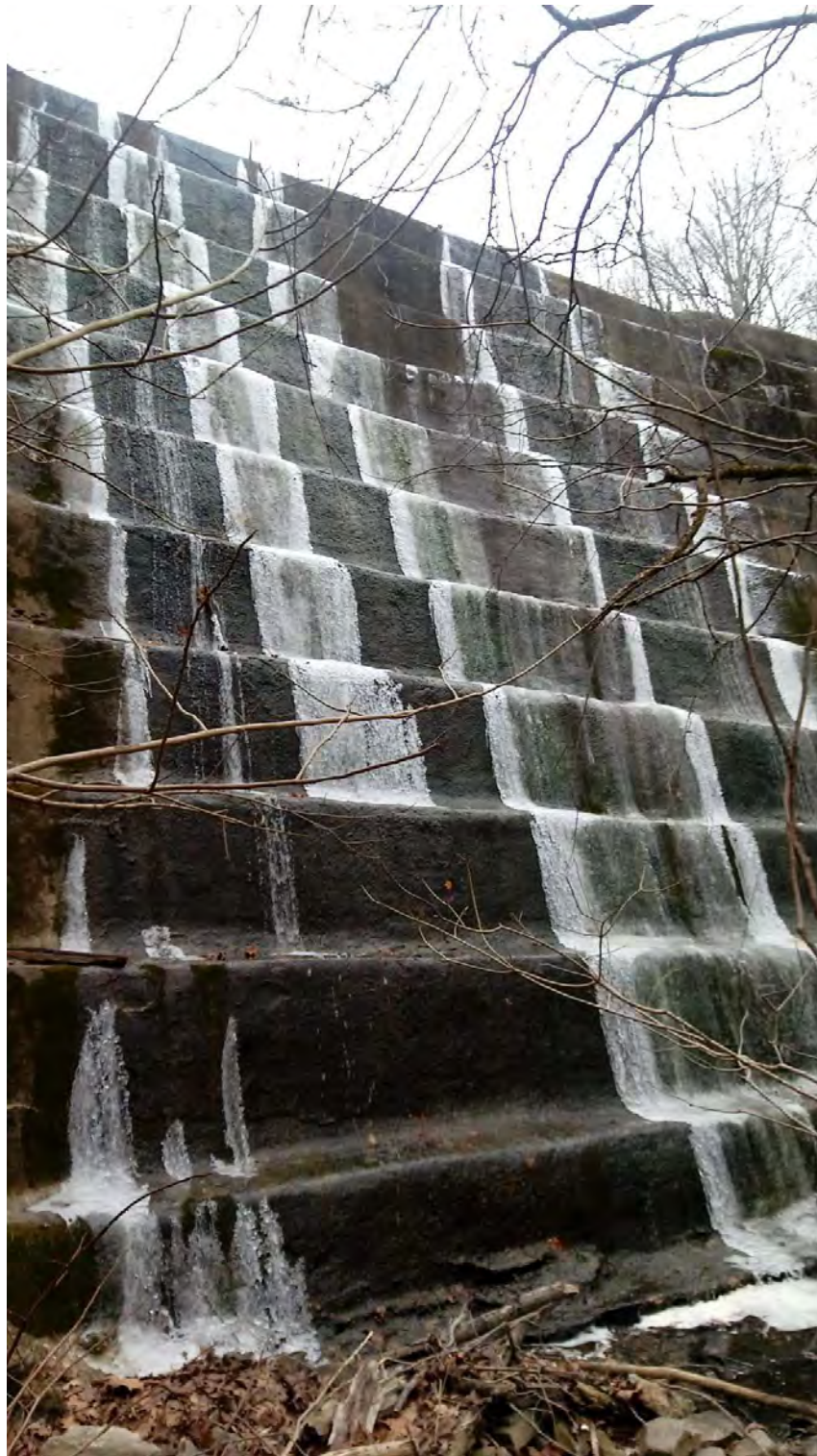
Figure 6. 1911 University Dam at University Lake from 12Mo1613 is a stepped arched dam made of concrete. View to south. Image courtesy of the Glenn A. Black Laboratory of Archaeology and the Trustees of Indiana University.
