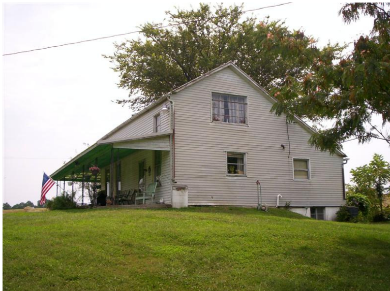
Figure 4. North and west façades of the Johnston House looking southeast. Photo from ThinkGIS (2017).
