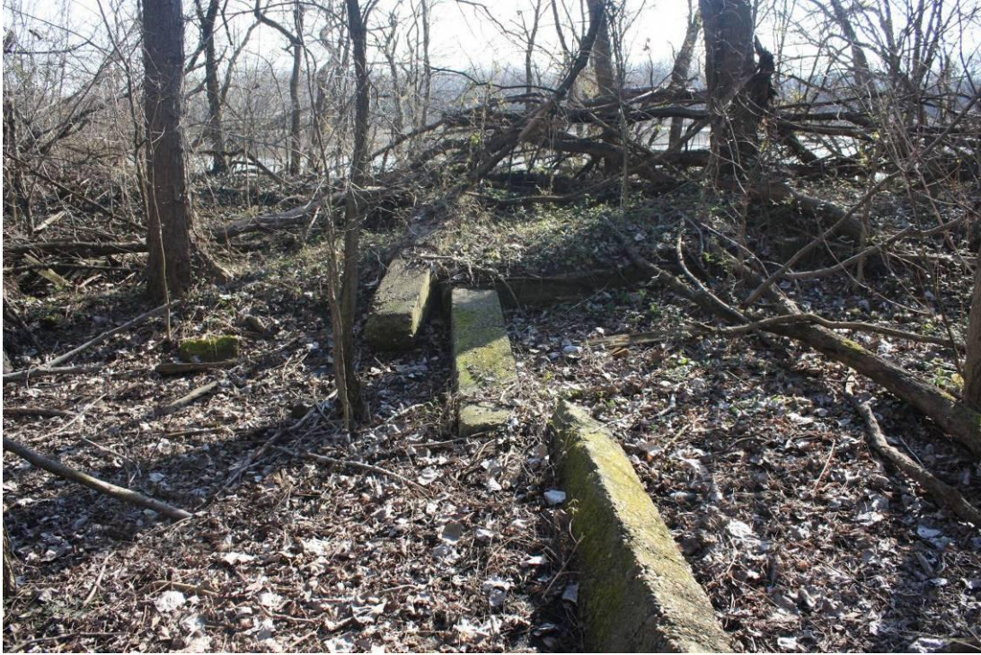
Figure 11. Concrete foundation posts (photo by Anne Tobbe Bader).
