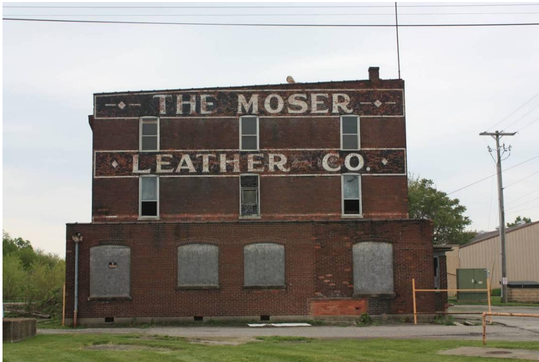
Figure 4. Westernmost tannery building with “THE MOSER LEATHER CO.”, facing southeast (photo by Anne Tobbe Bader).
