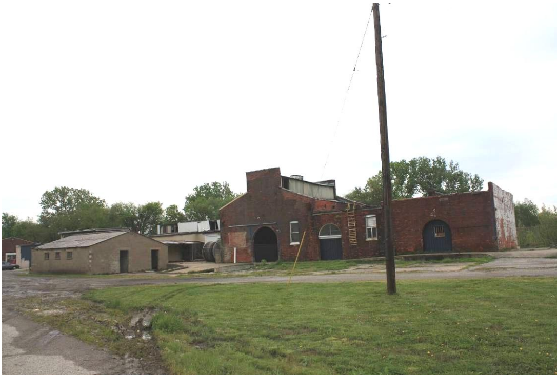
Figure 6. Additional vacant buildings at the tannery, facing southeast (photo by Anne Tobbe Bader).
