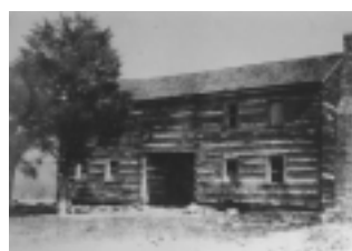
Granny White House at original location
