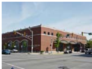
SAINT JOSEPH COUNTY PUBLIC LIBRARY 304 South Main Street • South Bend, IN 46601
