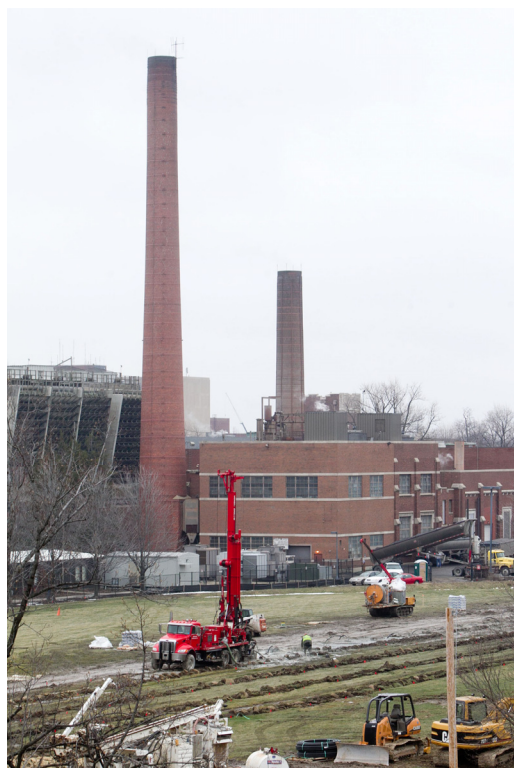
Bore Drilling for Geothermal Phase II
