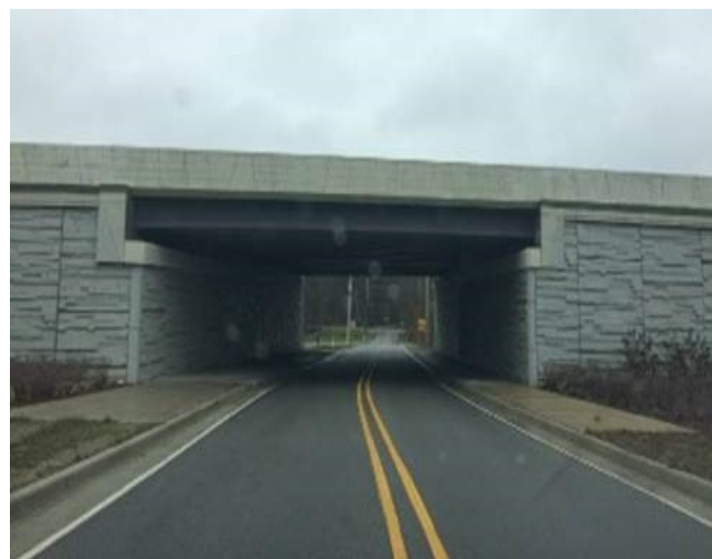
Figure 6-2: Elevated Freeway with Local Underpass – Mainline Option M1
