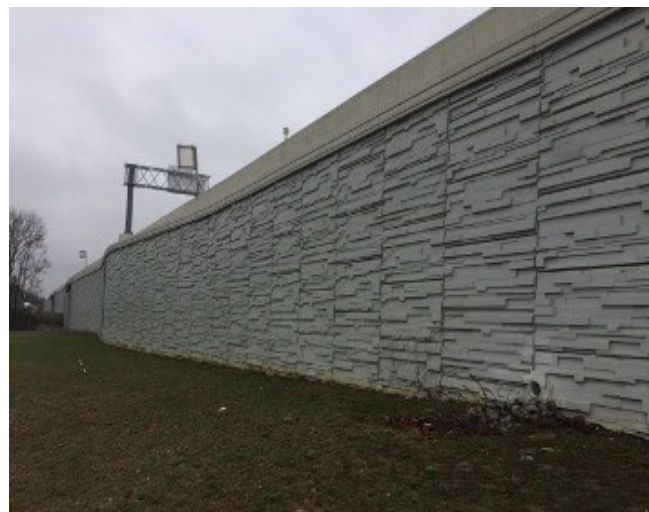
Figure 6-1: Typical Freeway Retaining Wall
