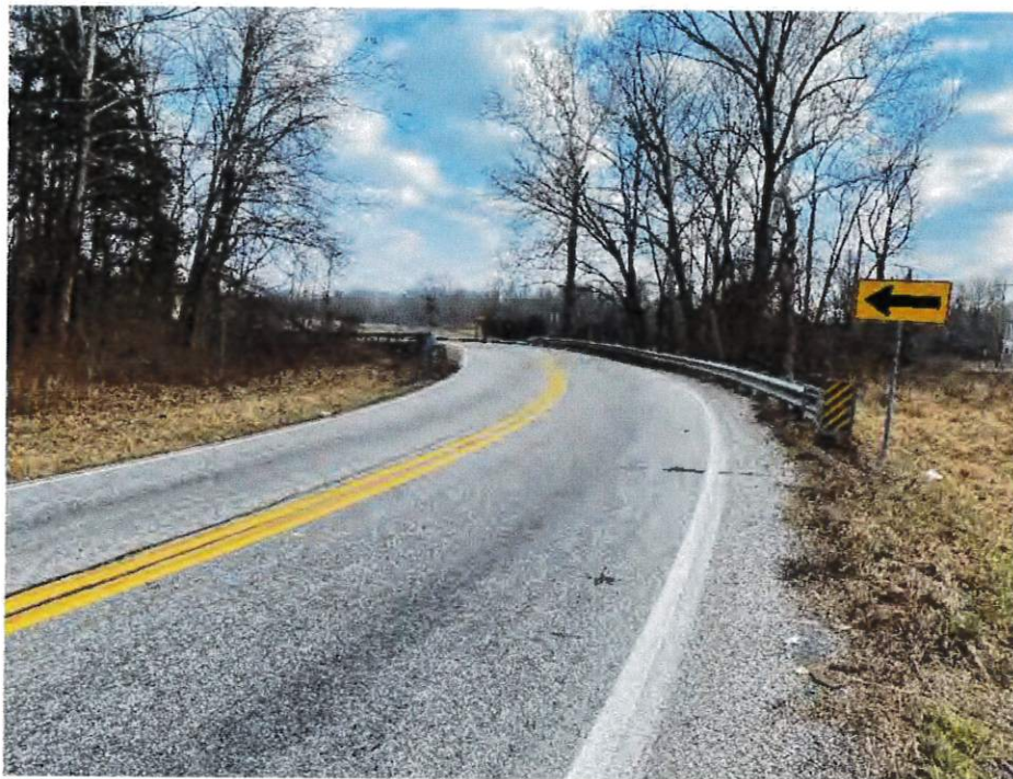
Photo 4. Streetscape view of Bridge No. 058-03-05882B carrying State Road 58 over White Creek facing northeast
