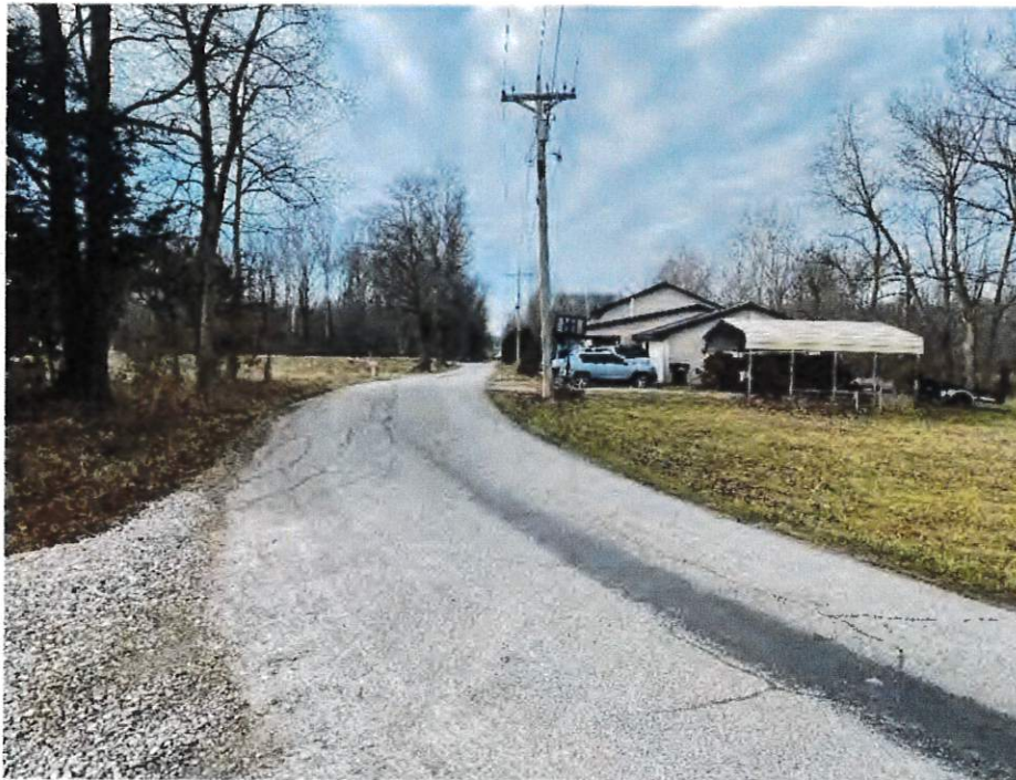
Photo 11. View of County Road 700 South showing 9550 West 700 South facing west from the east end of the APE
