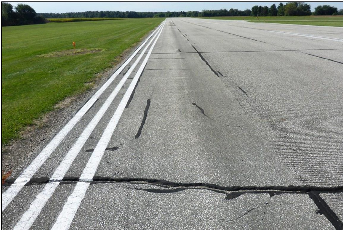
Figure 2-5. Typical AC Pavement in Fair Condition (Feature 5030)
