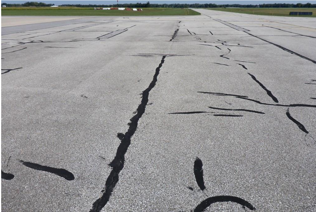
Figure 2-6. Typical AC Pavement in Poor Condition (Feature 3010)
