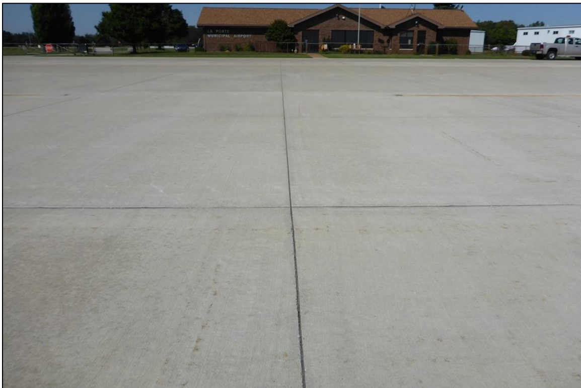
Figure 2-3. Typical PCC Pavement in Good Condition (Feature 3030)
