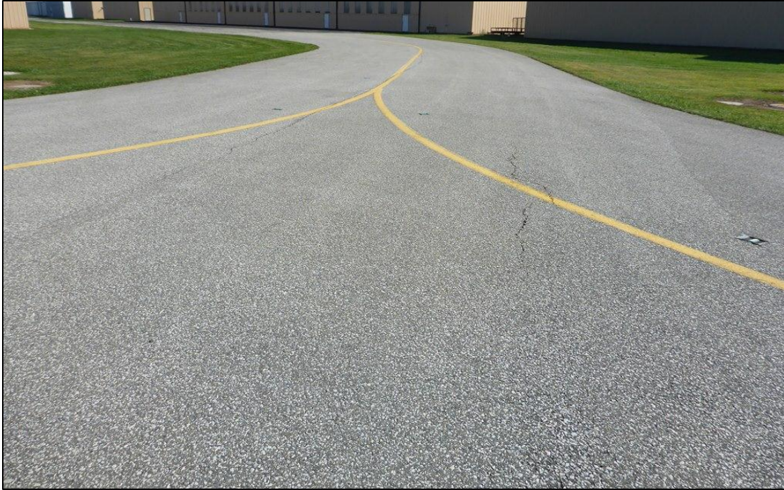
Figure 2-4. Typical AC Pavement in Good Condition (Feature 255)
