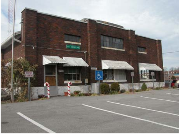
New Albany Subdistrict Garage. Designed by Vonnegut, Bohn and Mueller Architects, 1932.
