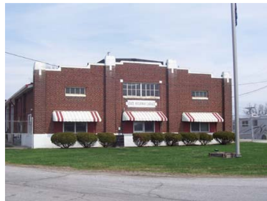
Tipton Subdistrict Garage
