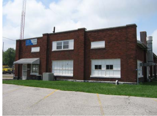
Evansville Subdistrict Garage. Designed by Vonnegut, Bohn and Mueller Architects? 1933.
