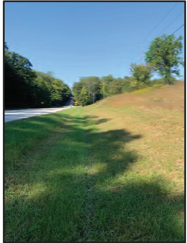
23. View of mowed ROW and RSD4 along the north side of SR 258, looking west. 9/28/2021
