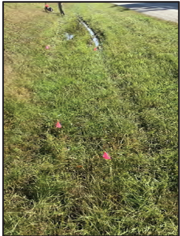
28. View of Wetland A, located within a roadside ditch along the north side of SR 258 and east of N CR 100 E, looking east. 9/28/2021
