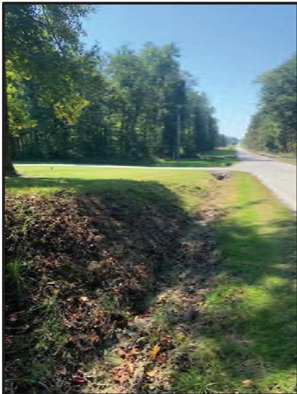
6. View of mowed ROW, RSD9, and driveway entrance along the south side of SR 258, looking west. 9/28/2021
