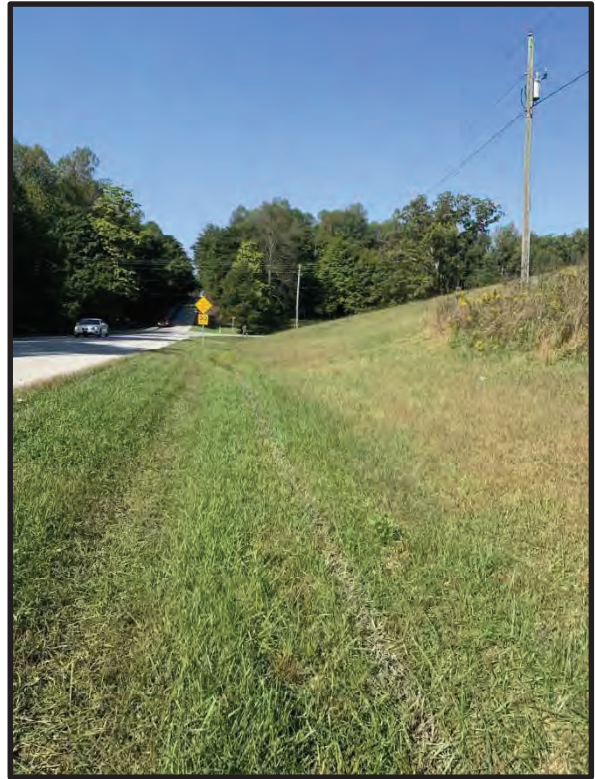
27. View of RSD4 into Wetland A, located north of SR 258, looking west. 9/28/2021
