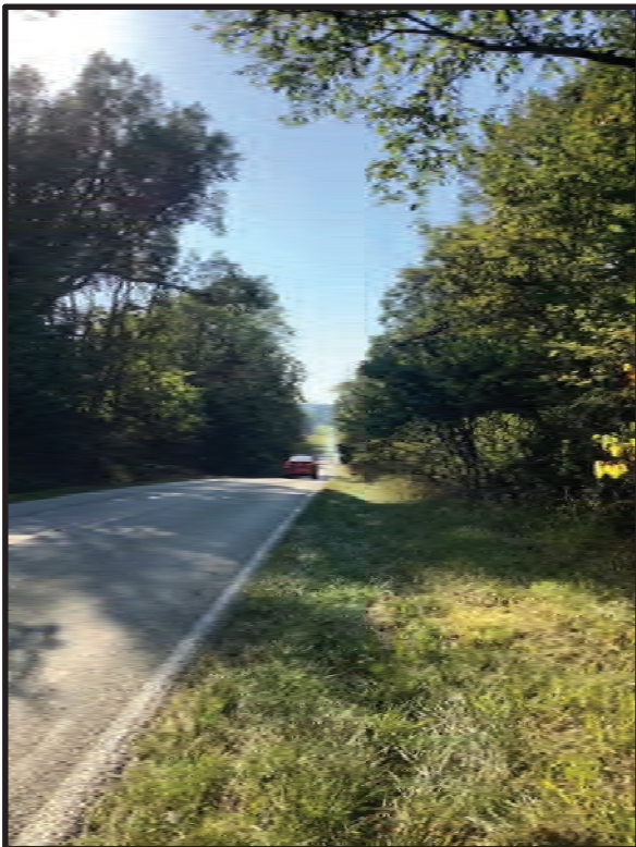
10. View of mowed ROW and upland forested area along the north side of SR 258, looking west. 9/28/2021
