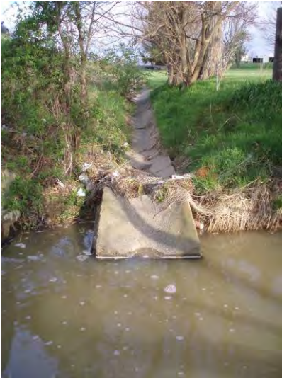
Photo 27. Structure E, UNT 5; east side of SR 60 facing northwest.
