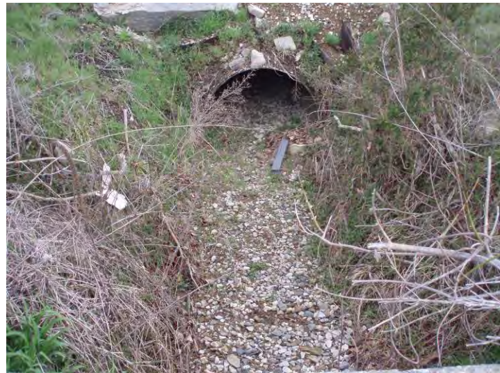
Photo 12. Structure C, UNT 3; north side of SR 60 facing northeast.
