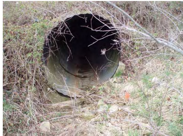
Photo 8. Structure B, UNT 2; north side of SR 60 facing pipe.
