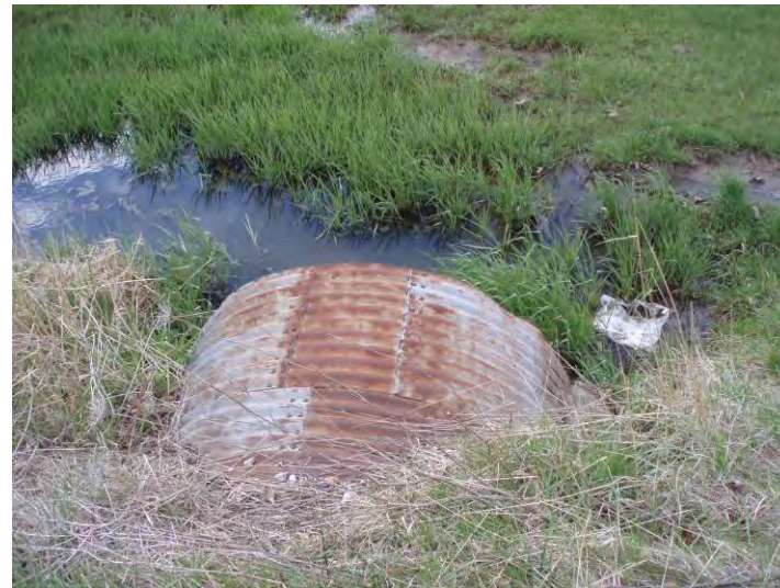
Photo 4. Structure A, UNT 1; south side of SR 60 at pipe.
