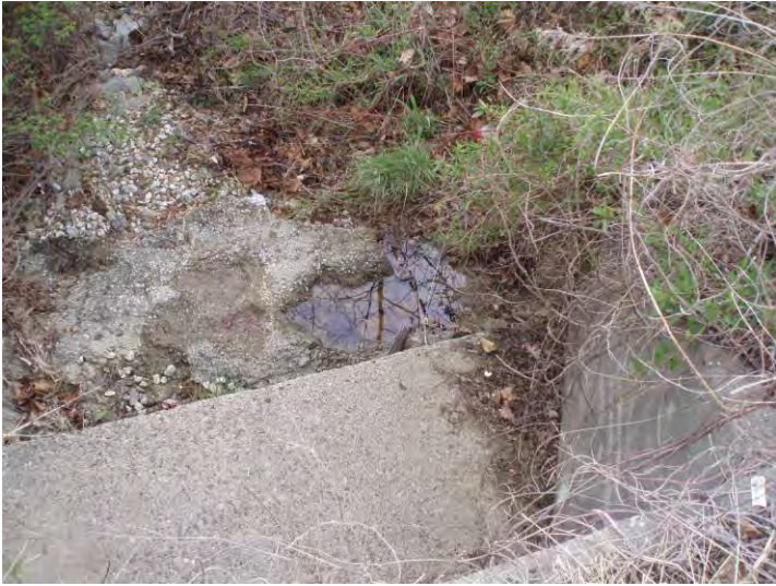
Photo 17. Structure C, UNT 3; south side of SR 60 looking down from structure.
