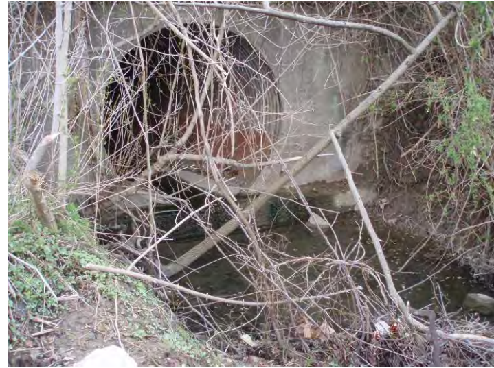
Photo 22. Structure D, UNT 4; south side of SR 60 facing pipe.
