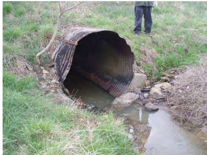
Photo 32. Structure E, UNT 5; west side of SR 60 facing pipe.
