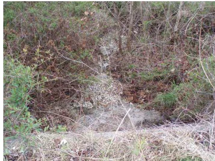
Photo 16. Structure C, UNT 3; south side of SR 60 facing southwest.
