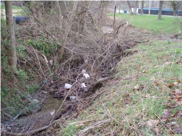
Photo 23. Structure D, UNT 4; south side of SR 60 facing south.
