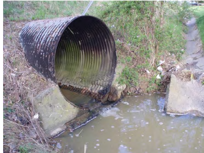
Photo 28. Structure E, UNT 5; east side of SR 60 facing pipe.
