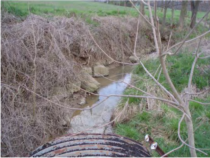
Photo 29. Structure E, UNT 5; west side of SR 60 facing west - southwest.
