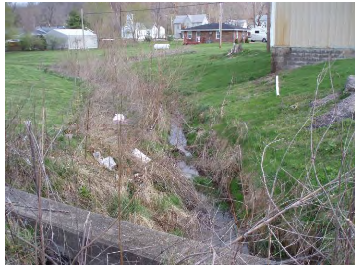
Photo 20. Structure D, UNT 4; north side of SR 60 facing north.
