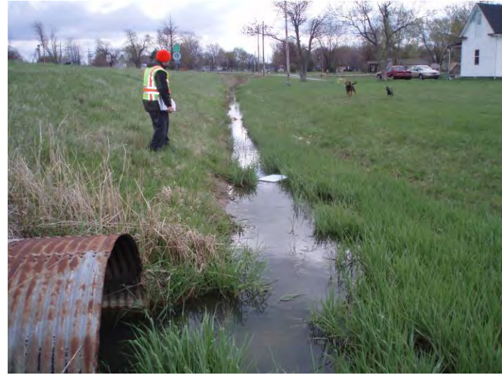
Photo 6. Structure A, UNT 1; south side of SR 60 facing east.
