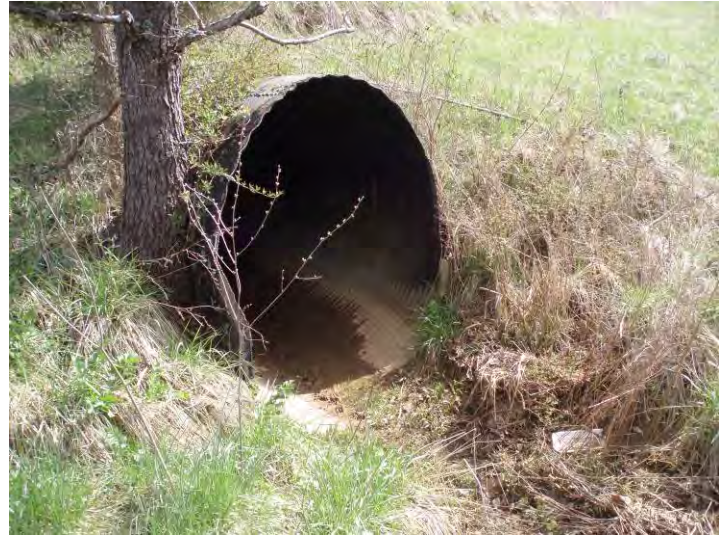
Photo 10. Structure B, UNT 2; south side of SR 60 facing pipe.
