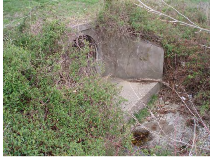
Photo 18. Structure C, UNT 3; south side of SR 60 facing pipe.
