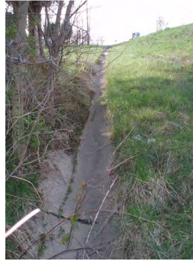
Photo 26. Structure E, UNT 5; east side of SR 60 facing southeast.
