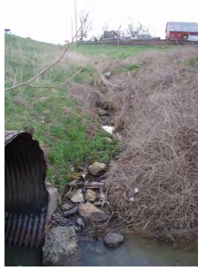
Photo 30. Structure E, UNT 5; west side of SR 60 facing southeast
