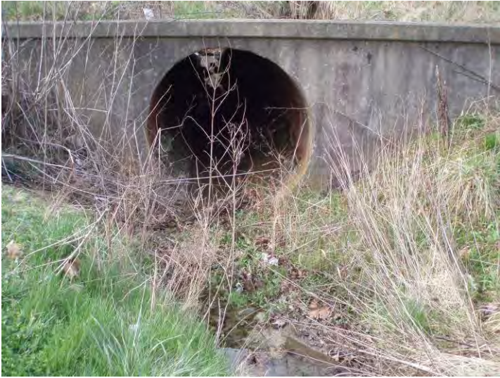
Photo 21. Structure D, UNT 4; north side of SR 60 facing pipe.
