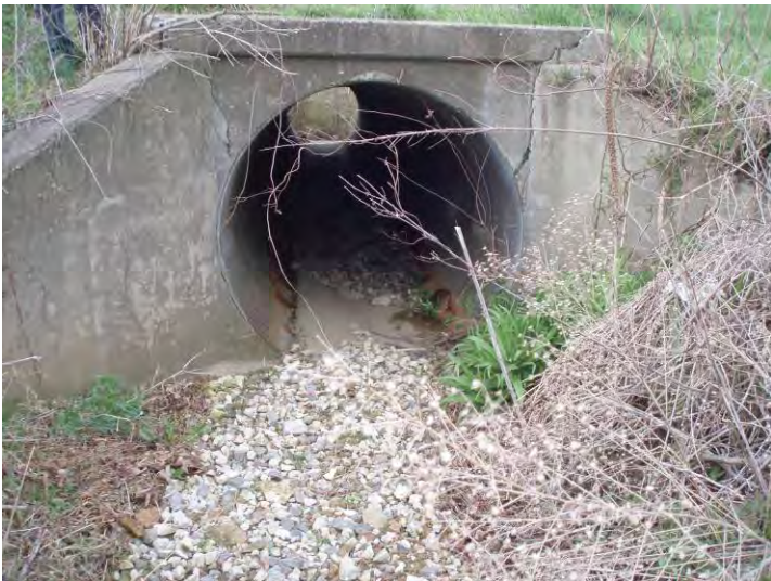
Photo 15. Structure C, UNT 3; north side of SR 60 facing pipe.
