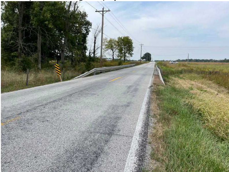
Photo 7. Facing west along the north side of SR 44, looking towards the project structure over UNT to Koots Fork.
