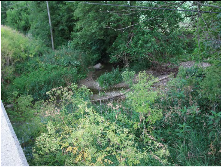
33. Looking northwest from the northeast quadrant of the bridge at the outfall of UNT to Mud Creek.
