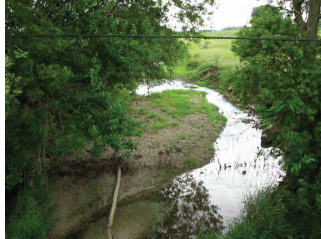
2. Looking north at Mud Creek from US 36 bridge over Mud Creek.
