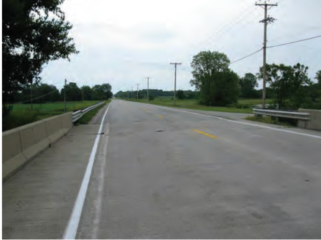
1. Looking east on US 36 from US 36 bridge over Mud Creek.
