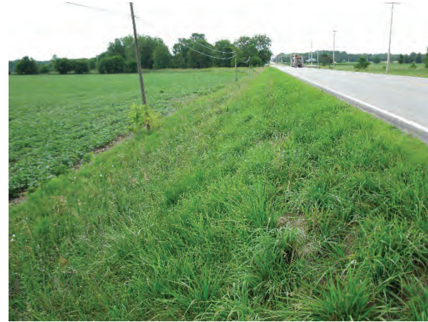
10. Northeast project quadrant, looking east.
