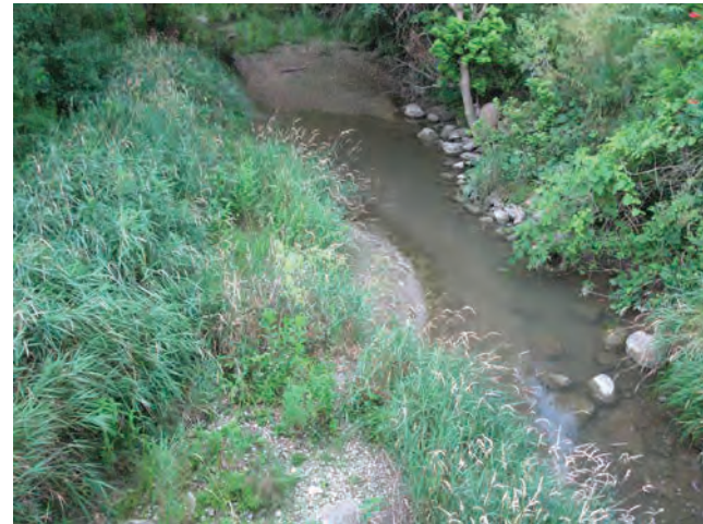
4. Looking south at Mud Creek from US 36 bridge over Mud Creek.
