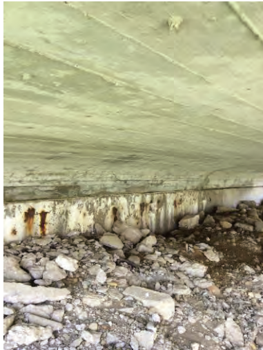
7. US 36 bridge span underside over Mud Creek.
