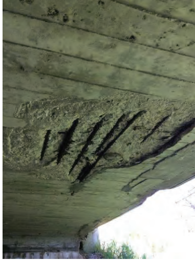
5. US 36 bridge span underside over Mud Creek.
