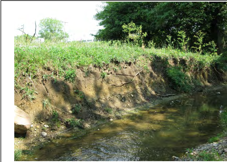
9. Looking southeast at the east bank scour of Mud Creek, north of the bridge.
