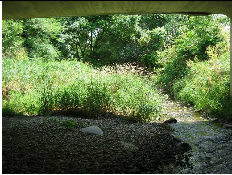
6. Looking south in Mud Creek from under the bridge. Note the instream wetland feature on left side.
