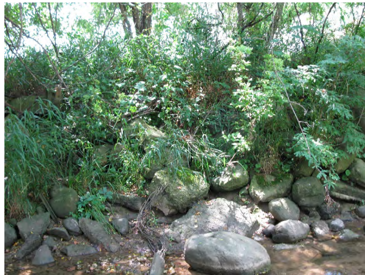
4. Looking at west bank of Mud Creek, south of bridge.
