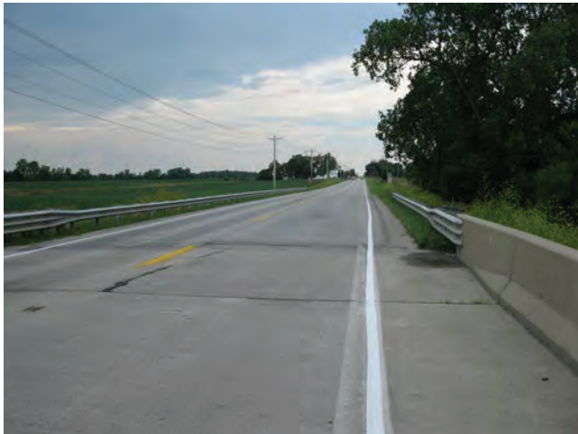
3. Looking west on US 36 from US 36 bridge over Mud Creek.
