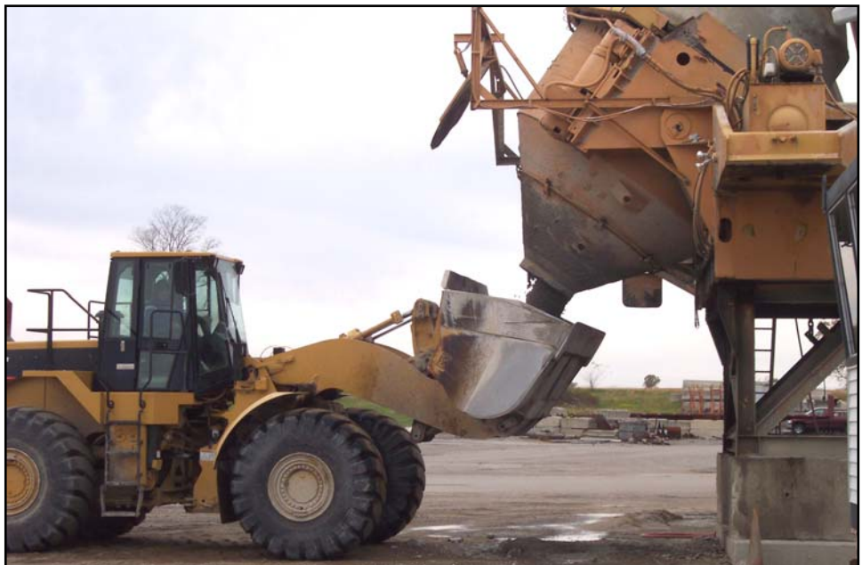
Figure 3-6. Loading a Bucket
