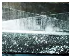
DUCT CONDENSATION
