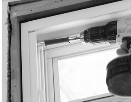
Block frame window installation: Block-frame windows don't have a
