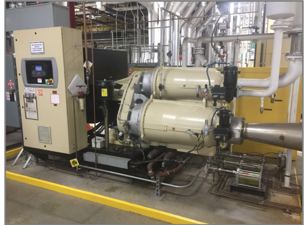
Photo 1: Before - 500 hp Centac Air Compressor
