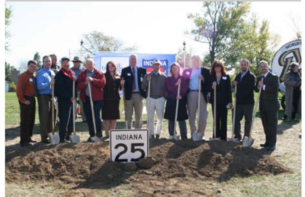
October 22, 2008— Governor Daniels helped break ground on the Hoosier Heartland Highway in Lafayette..
