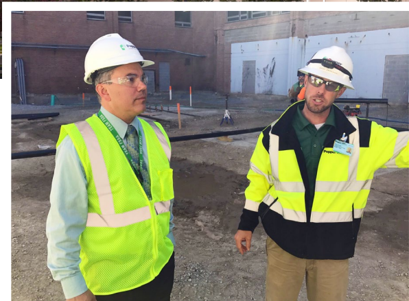
Eric Zeronik from Pepper Construction (right) gives Mark Newell, deputy director, State Psychiatric Hospitals, a tour of the site.
