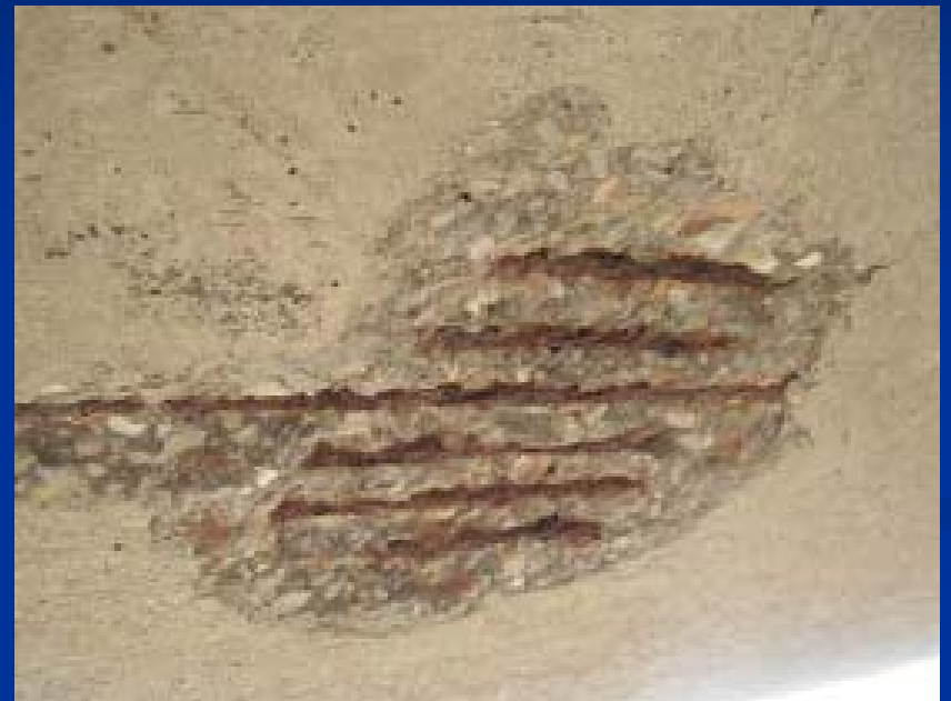
Corrosion Damage
