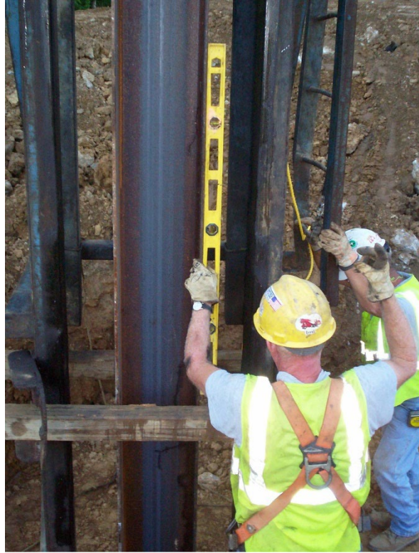
Figure 11 Contractor Checking Pile Alignment
