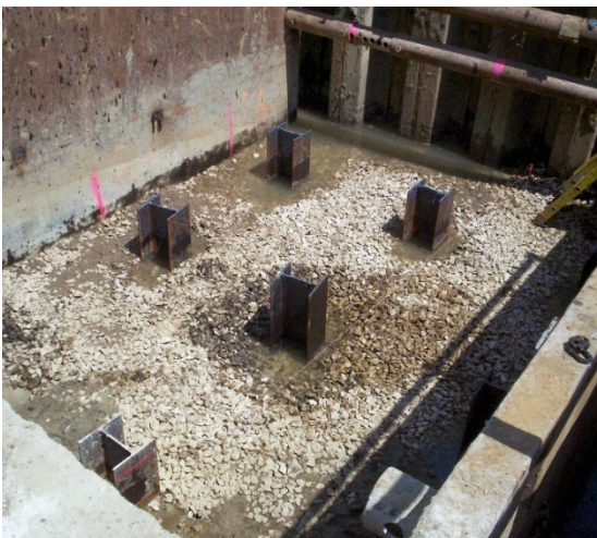
Figure 14. Piles cut-off at plan elevation
