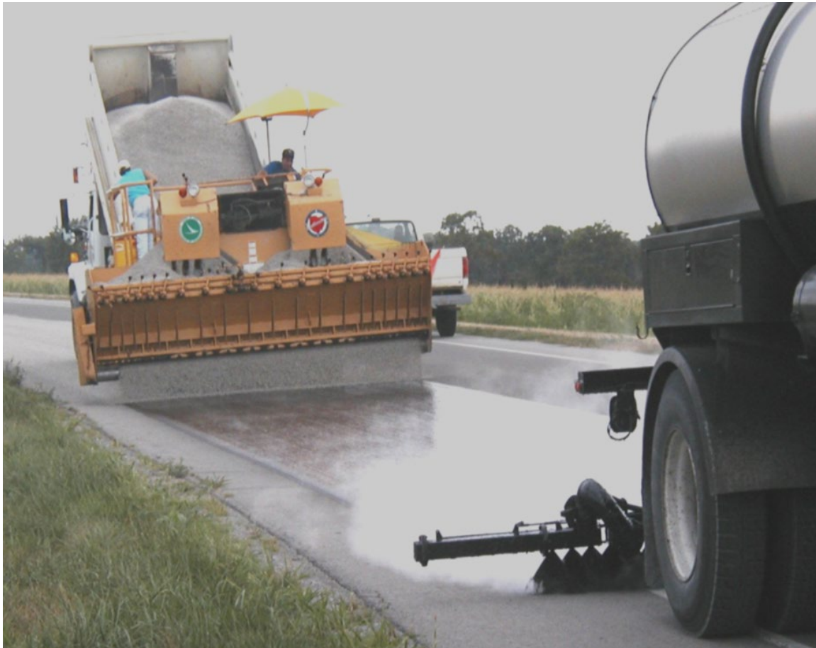
Figure 13.24-11 Aggregate Spreader
