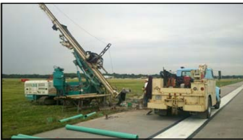
Above: Drilling an angled borehole. Below: Introducing grout into a hole.
