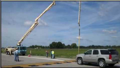
Above: Drilling an angled borehole. Below: Introducing grout into a hole.
