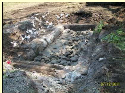
Flowable fill covers the aggregate.
