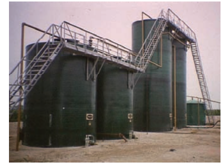
Crude Oil Tank Battery
