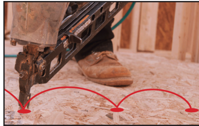
Bump firing is using a nail gun with a contact trigger held squeezed and bumping or bouncing the tool along the work piece to fire nails. (Photo illustration from federal OSHA publication.)
